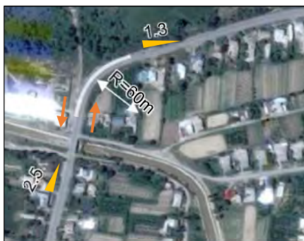
Figure 2-2-22 Existing Road Condition near the 83 km Post
