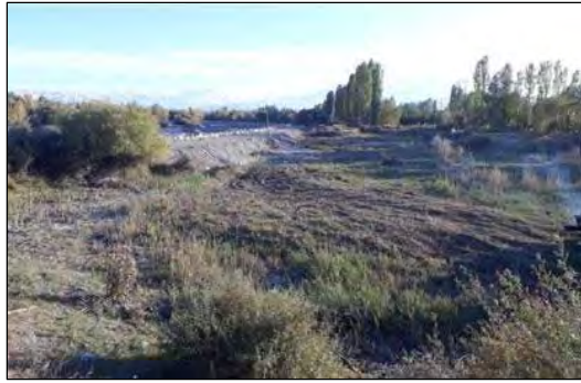
A: River Bank in the Area of Drilling Works
