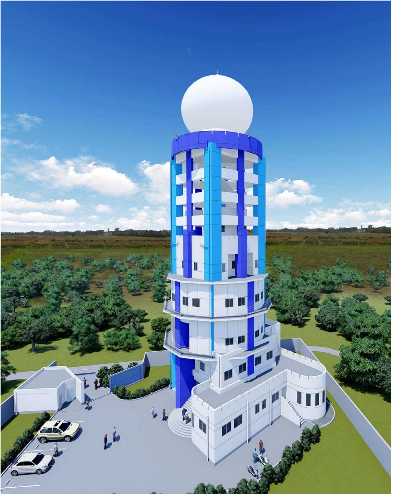
Multan Meteorological Radar Tower Building
