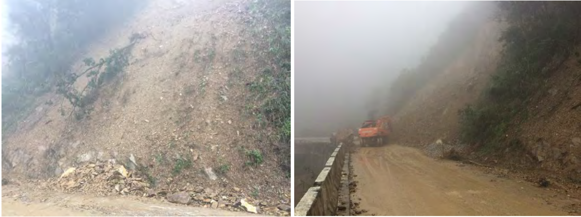
Figure 8.2.9 Slope Failures Generated around Border on National Road No.8
