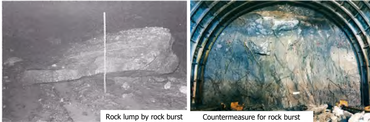
Figure 5.4.3 Rock Burst during Construction of Kan-etsu Tunnel
