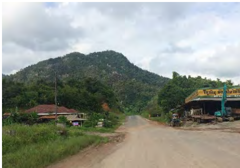
Simple Pavement Section (8 km from Viengthong)
