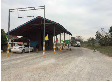
Vehicle Weight Estimation Facility at Laksao (NR 8)
