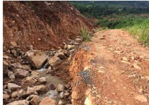
After 8 km from Viengthong, the road condition has deteriorated in the rainy season for several years after the suspension of the construction
