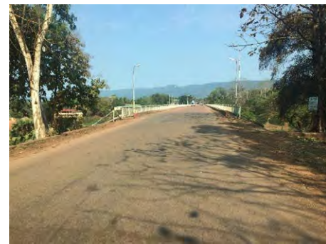
Suburb Area (2 Lanes for Road and Bridge Section)
