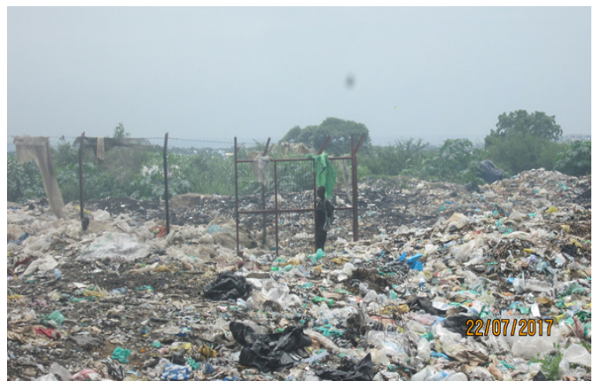
Image 3-24 Surrounding fence was broken
