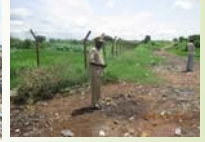
Director of Rejaf Payam inspecting what remains of the fence.
