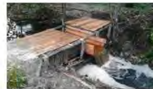
Figure 16. Canal Blockage for Rewetting Peatland
