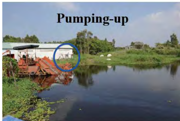
Fig. 20b. Water pumping-up from the river side
