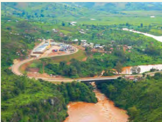
Rusumo International Bridge and OSBP facilities on the Tanzania-Rwanda border
