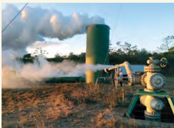
Geothermal well testing
