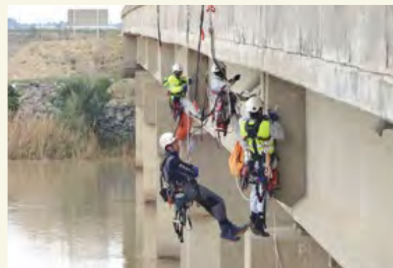
ADM personnel training held at a bridge in Morocco
