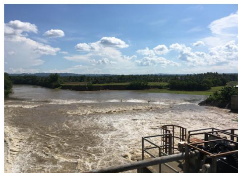
⑭ Pagalungan diversion dam (water and trees) (W:S:V=5:1:1 • 1:2:5, Linandangan@18/06/2017)
