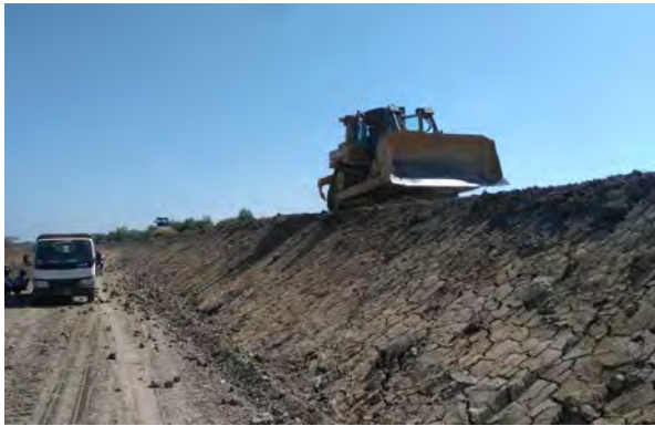
An example of dike constructed in a polder area, height ranges from 3 to 3.5 m.
