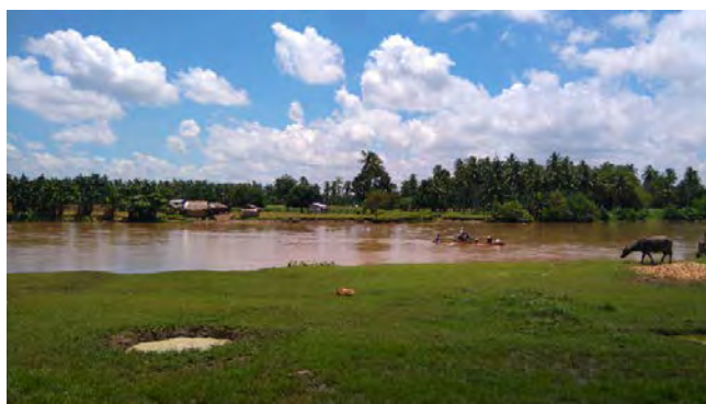
The location where PMC goes crossing the Pulangi River through a siphon structure (box size: 1.3m x 1.3m, length: 141 m).
