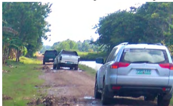
The picture shows service road along the main canal in the Maridagao Service Area. Some parts of earthen road become muddy due to rain.
