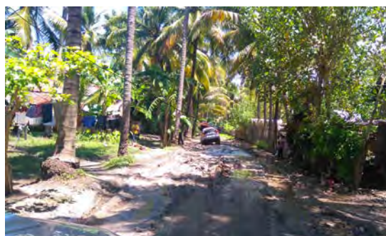
A typical Barangay Road in LMSA, becoming hardly passable during rainy season
