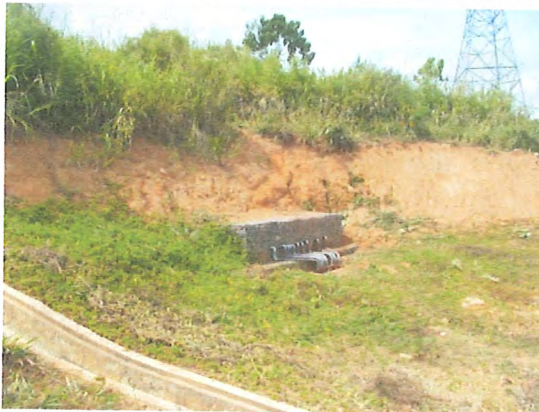
Photo 11: Soils have been removed (D.P.6)
