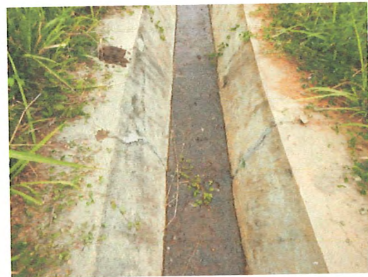
Photo 4: Cracks have been corrected (Loc.5)
