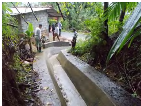
Photo 11: Additional wall for the overflowing has been constructed. (Loc. 14)
