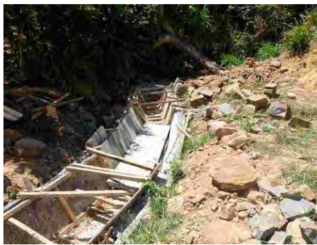
Photo 4.4 Sudden curves of ditch (already corrected )
