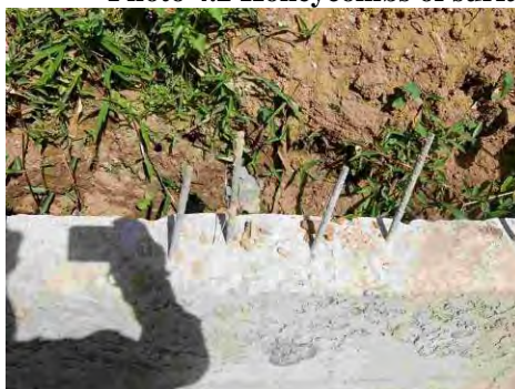
Photo 4.3 Spacing of steel bars do not follow the design (already corrected)
