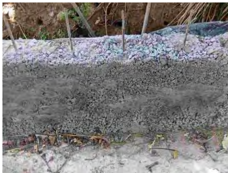
Photo 4.2 Honeycombs of surface drainage ditch (already corrected)
