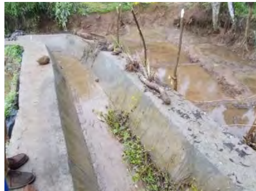
Photo 2: Leakages have been repaired.(Loc. 2)
