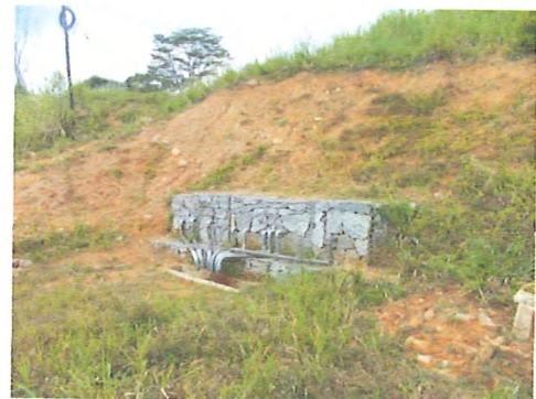
Photo 10: The small slip has been reshaped (D.P.4)
