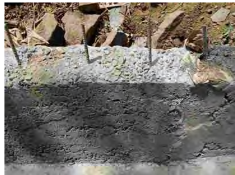
Photo 4.2 Honeycombs of surface drainage ditch (already corrected)
