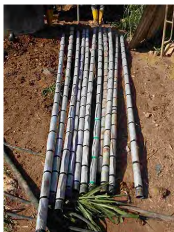
Photo 4.7 Wrapping of geotextile to PVC pipes (left: improper wrapping, right: proper wrapping)
