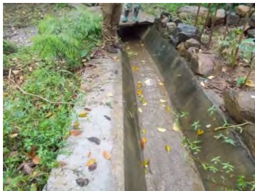
Photo 1: Crack on the ditch has been corrected. (Loc. 1)
