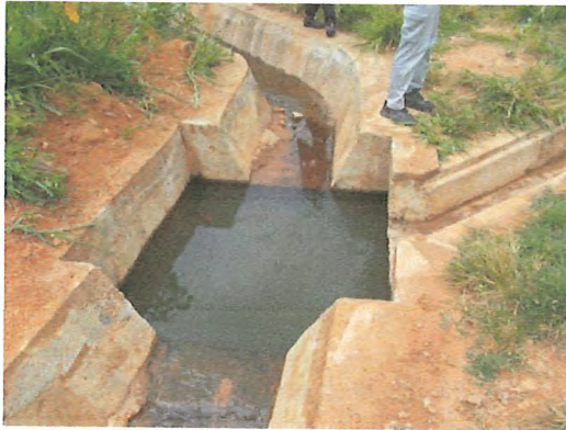
Photo 7: Soils have been removed (Loc.8)
