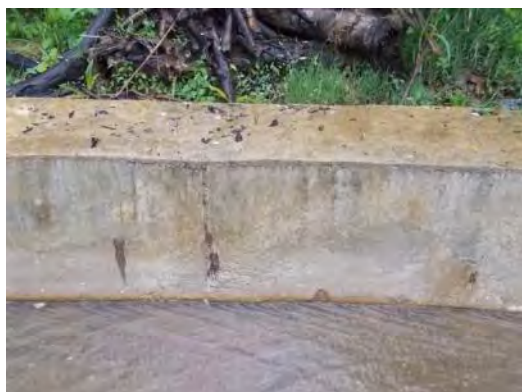
Photo 9: Leakage has been repaired. (Loc. 13)
