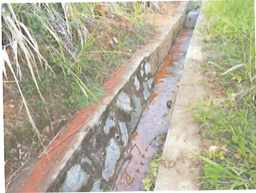
Photo 1: Erosion has been corrected (Loc.2)
