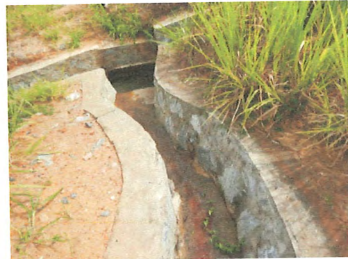
Photo 2: Erosion has been corrected (Loc.1)
