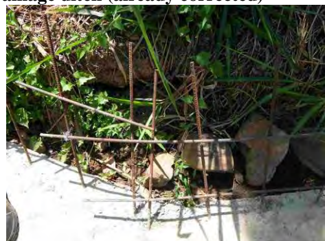
Photo 4.3 Spacing of steel bars do not follow the design (already corrected)
