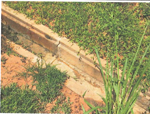
Photo 9: Crack has been corrected (Loc.11)
