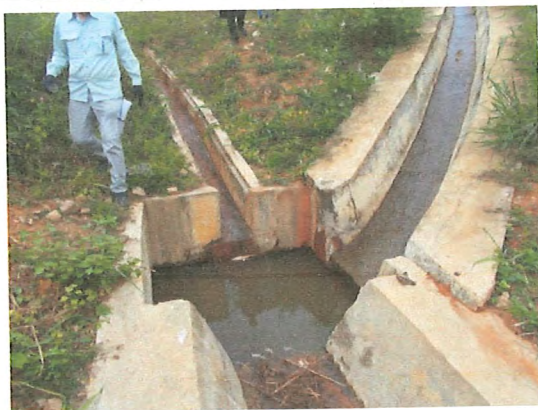
Photo 5: Soils have been removed (Loc.7)
