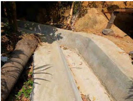
Photo 4.5 Sudden curves of ditch
