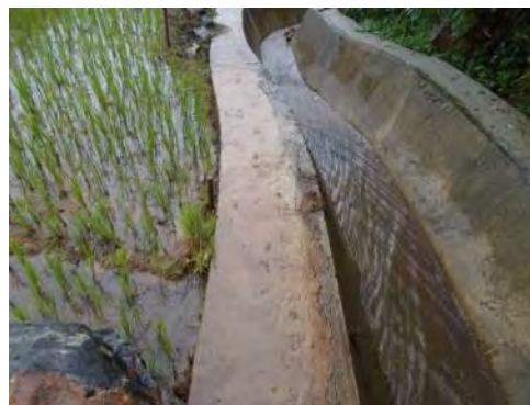
Photo 6: Crack has been corrected. (Loc. 5)
