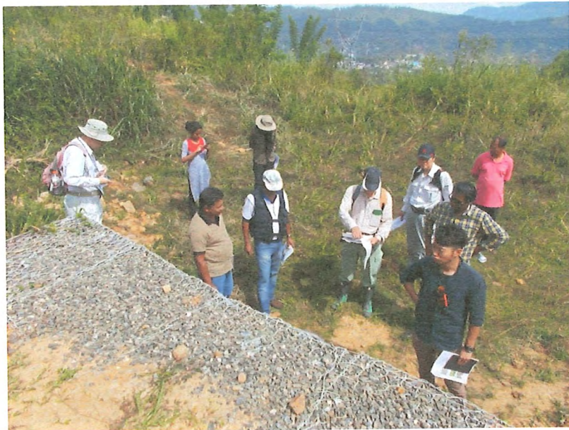
Defect Liability Inspection at the site
