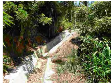
Photo 4.5 Sudden curves of ditch
