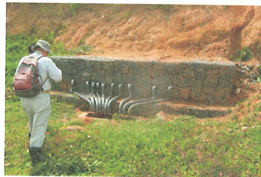
Photo 12: PVC pipe has been repaired (D.P.6)
