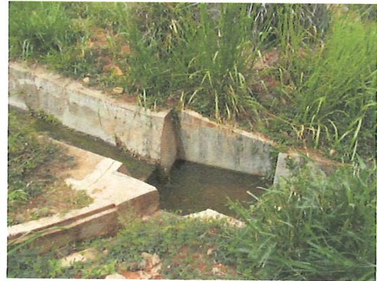
Photo 8: Soils have been removed (Loc.9)
