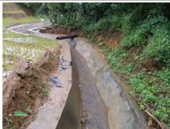
Photo 4: Leakages have been repaired.(Loc. 10)
