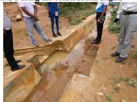
Photo 4.6 After the construction Pits are filled by soils
