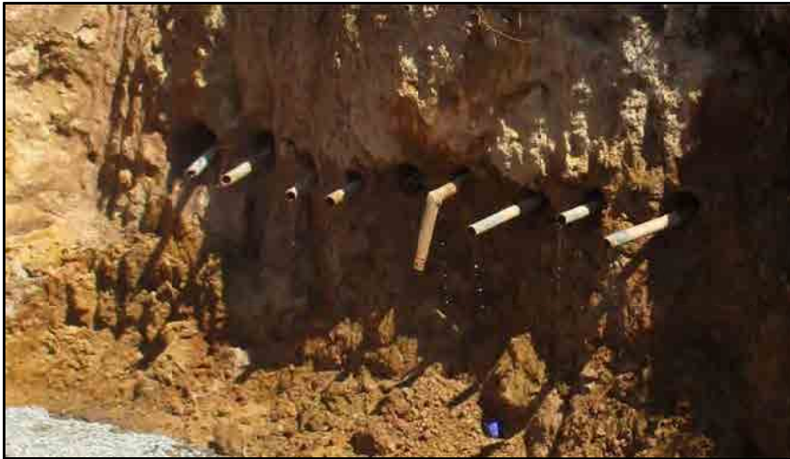
Drilling completed at location 5
