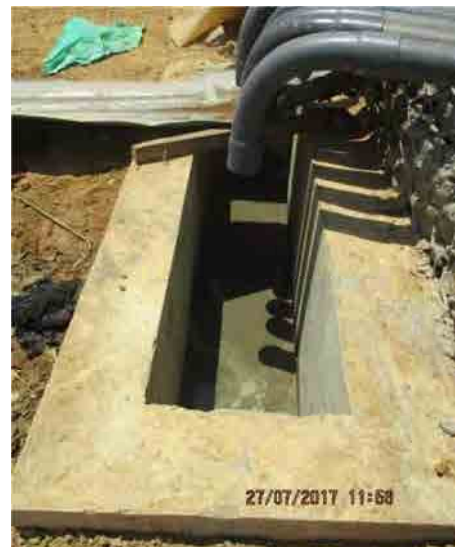
Type 1 catch pit constructed at location 4
