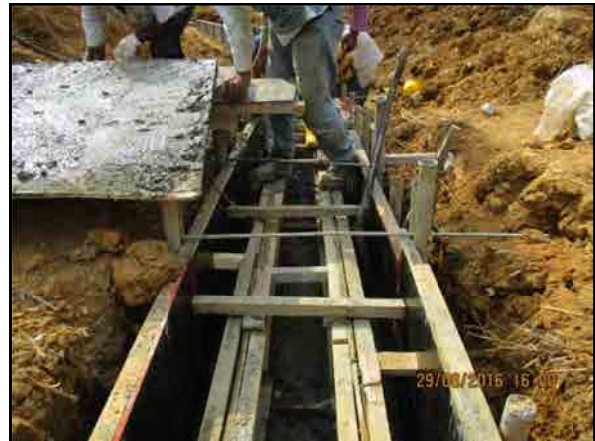
Formwork for concrete drains
