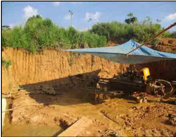
Holes being drilled at location 6
