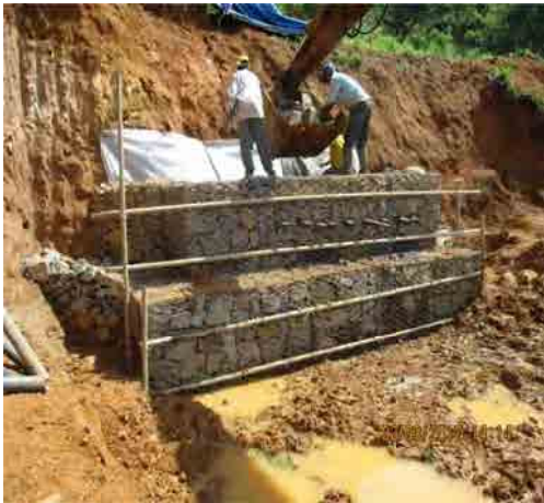
Gabion work at point location 6
