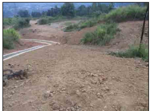
Reshaping around surface drains
