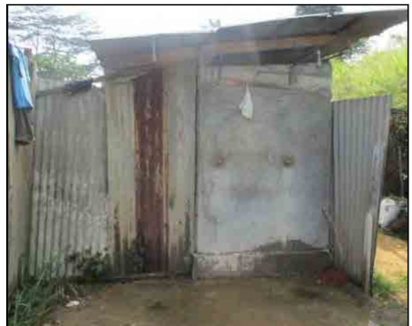
Bathing and washing facility at site
