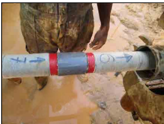
PVC pipes driven into holes through casing
