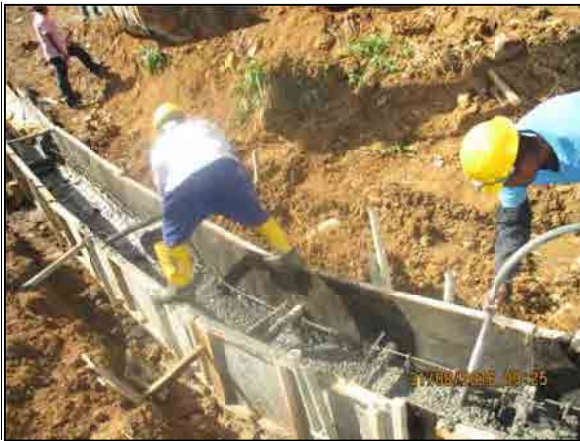
Formwork for concrete drains
