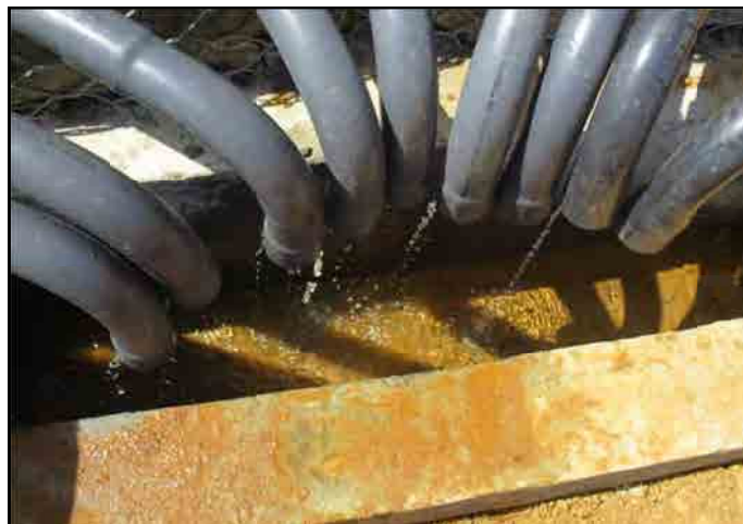
Drilling completed and PVC pipes routed to catch pit at location 4
