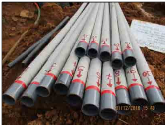
PVC pipes numbered before installation
