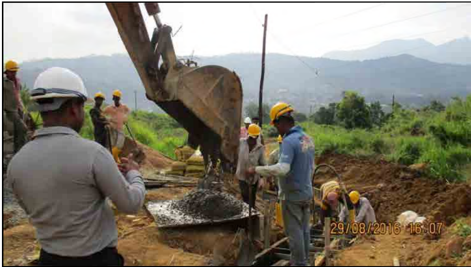
Concreting the surface drains
