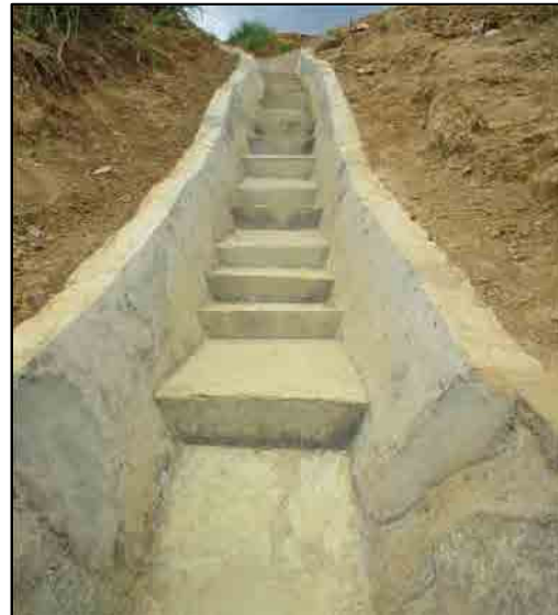
Additional cut off drain
