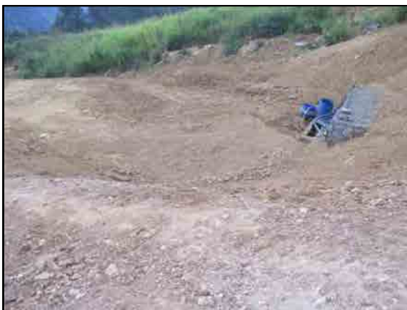
Reshaping completed at new location 4
