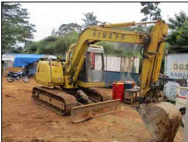
Laboratory, storage facilities, excavator at site
