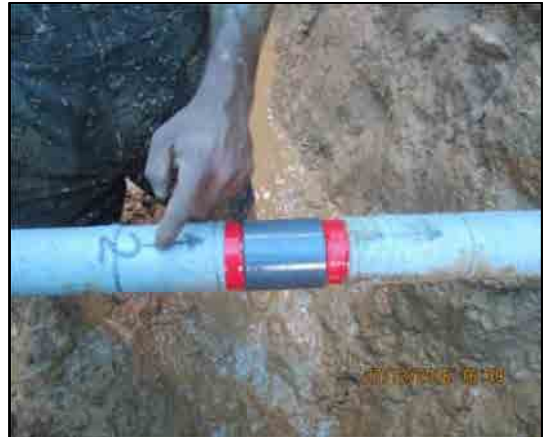
PVC pipes being installed in order
