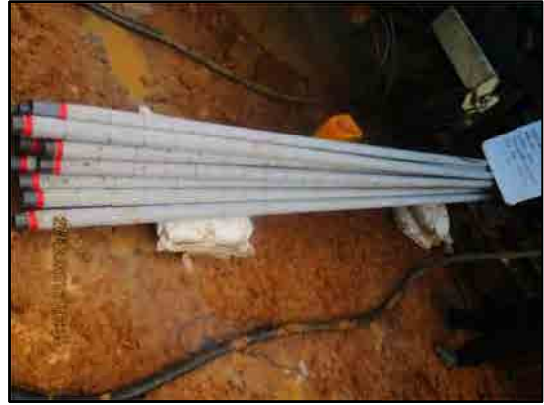
PVC pipes prepared and numbered before installation
