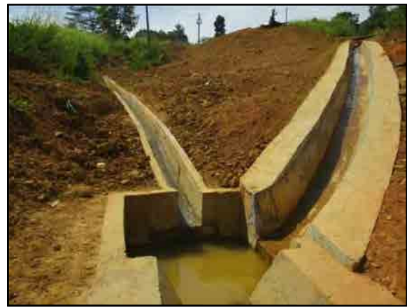
Type E, D and C drains joining together
