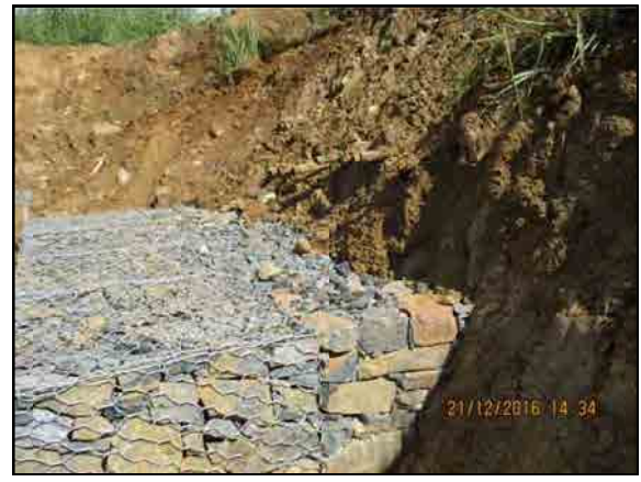
Stone filling behind gabion walls
