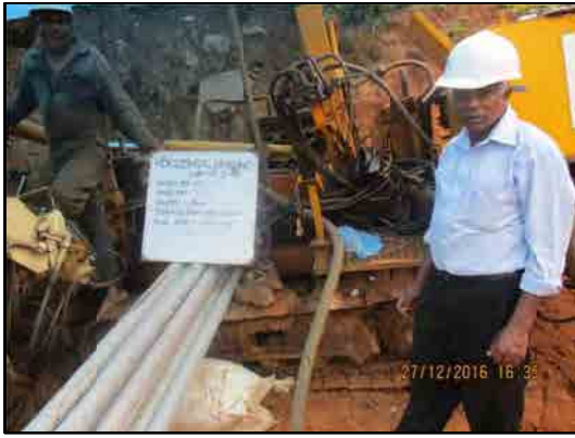
PVC pipes prepared and numbered before installation
