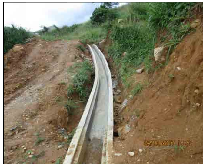
Neat and smooth finish of the drain
