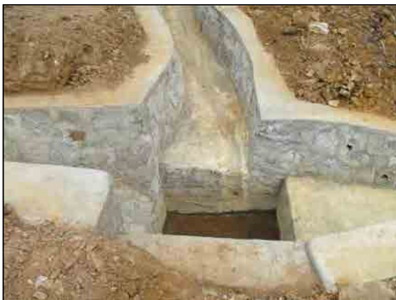
Drains additionally constructed
