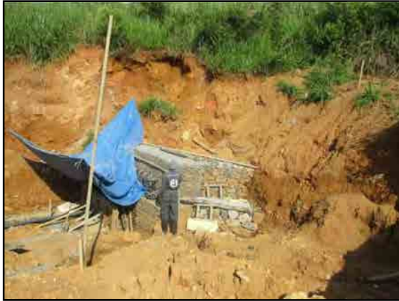
Stone filling behind gabion walls
