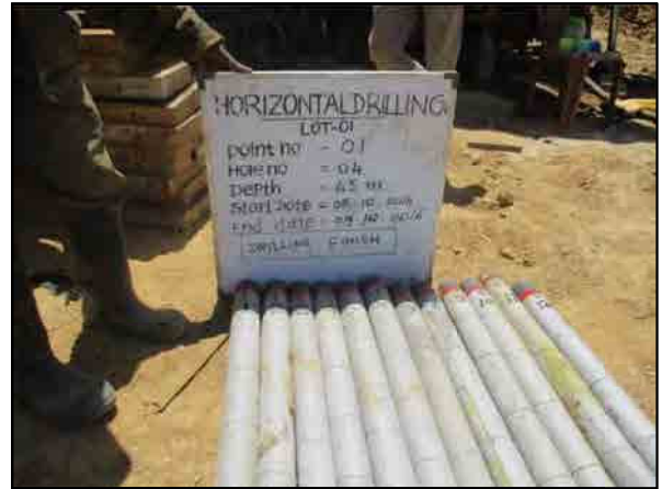
PVC pipes with geotextile cloth wrapped before installation
