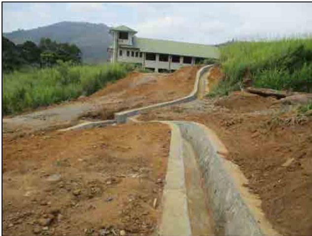
Additional cut off drain
