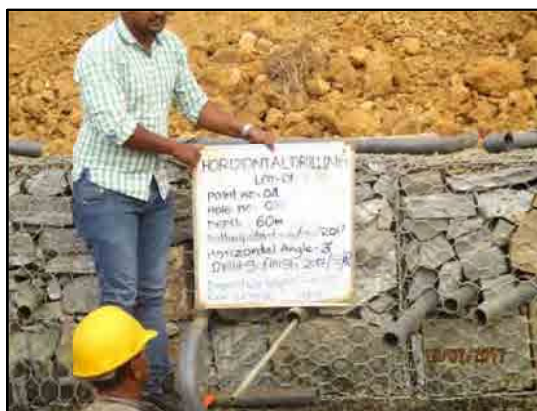
Hole lengths and Gabion work being measured and checked by JICA
