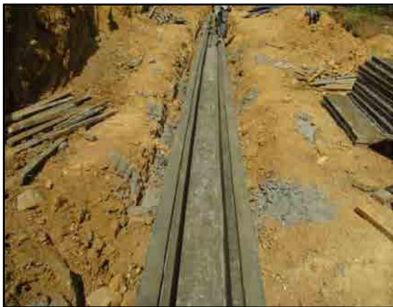
Type E drain when formwork removed
