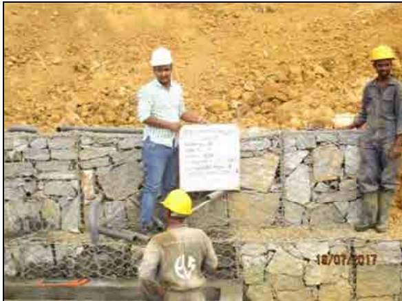
Horizontal drainage work being measured by JICA
