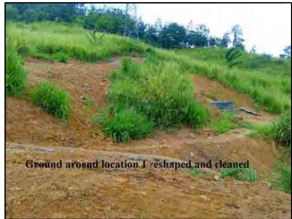
Location 1 after reshaping
