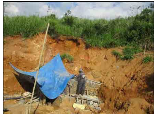
Stone filling behind and beside gabion wall
