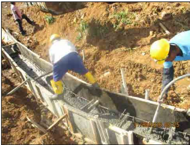
Concrete compacted with poker vibrator
