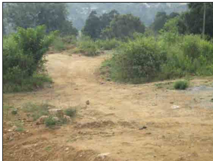
Temporary roads for construction
