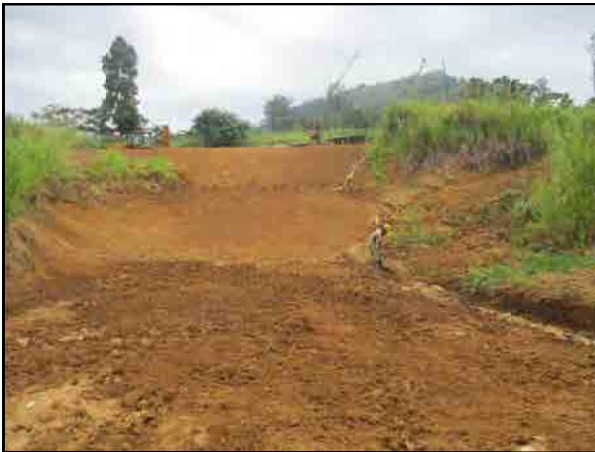
Old location 4 after reshaping
