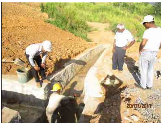
Inspection of additional drains by NBRO
