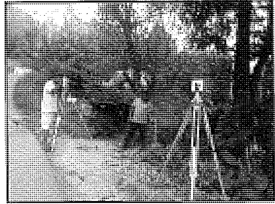
Fig 02: Pre surveying work
