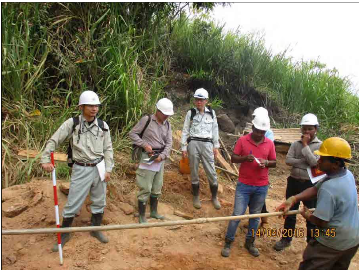
Checking the hole lengths at point 3 by JICA
