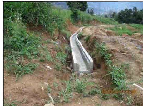
Type E drain (141m) starting point
