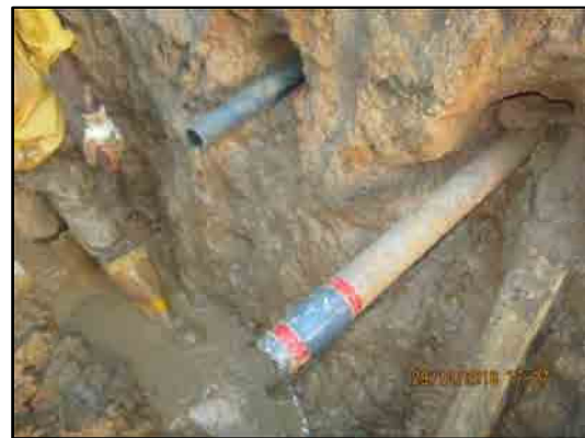
PVC pipes installed in to holes
