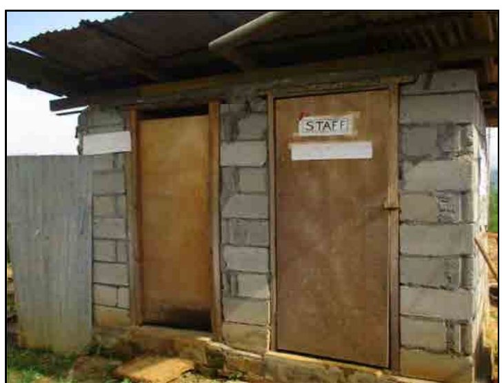
Sanitary facilities at site
