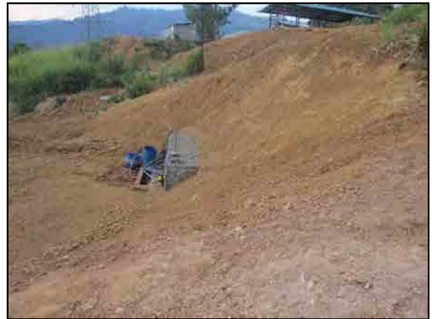
New location 4 after reshaping
