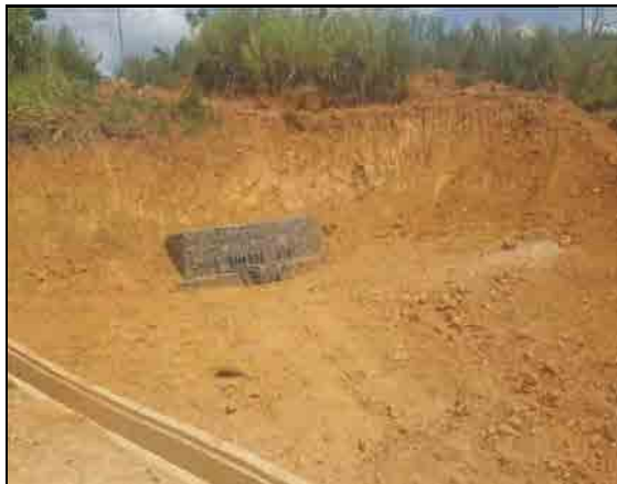
Gabion work at location 5
