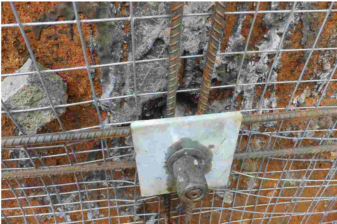
Photo 2 Example of soil nailing in Diyatawala (Source: TCLMP)
