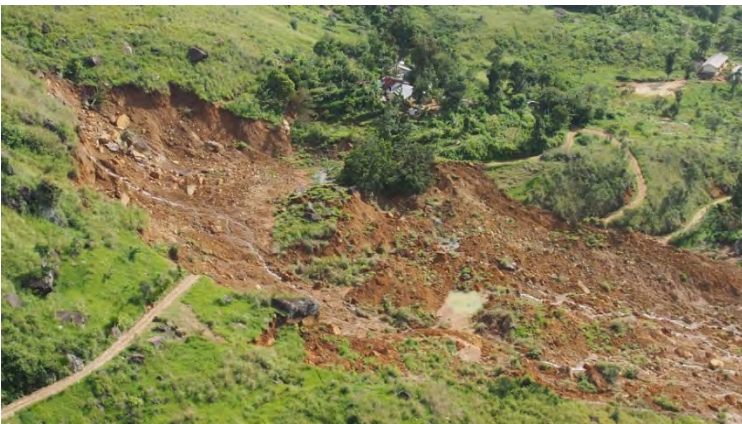
Scarp Condition of the Landslide Mass Remains
