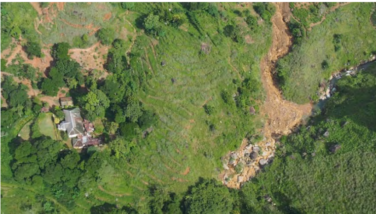
Landslide Mass Flowing in to the Stream
