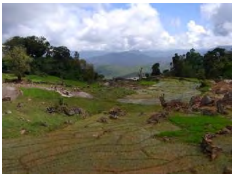
Close view of the lower slope of landslide
