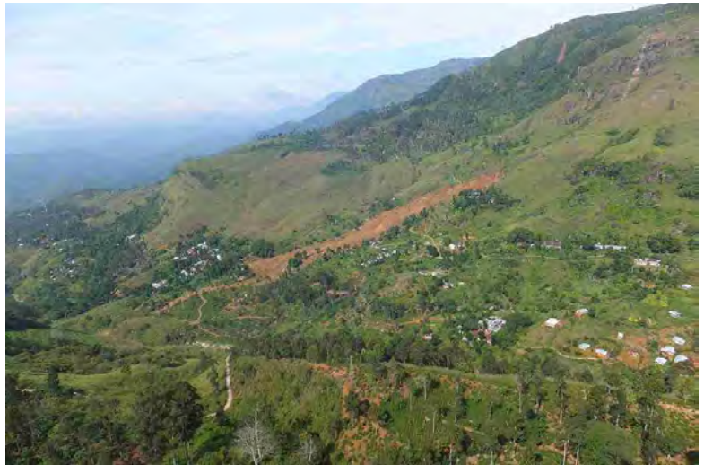
Photo-2 Angle of Landslide Slope
