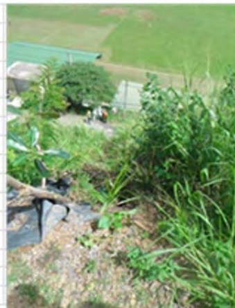
View of the lower slope from vestibule of the Nursing School
