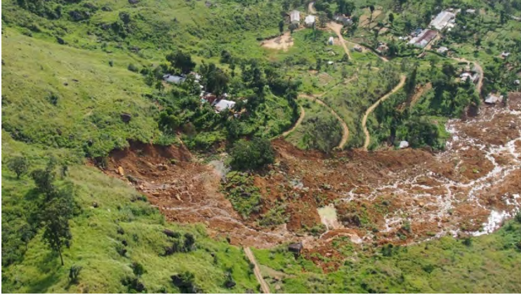
Water Flow at the head of the Landslide
