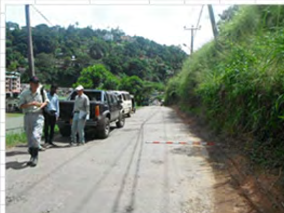
Road along the foot of the lower slope
