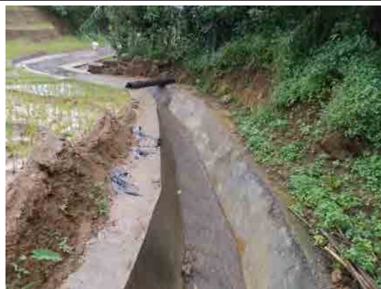
Photo 4: Leakages have been repaired.(Loc. 10)
