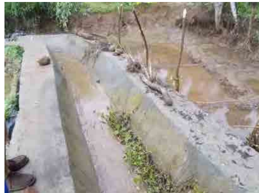
Photo 2: Leakages have been repaired.(Loc. 2)
