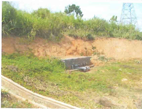
Photo 11: Soils have been removed (D.P.6)
