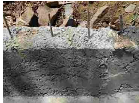
Photo 4.2 Honeycombs of surface drainage ditch (already corrected)
