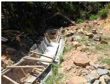
Photo 4.4 Sudden curves of ditch (already corrected )
