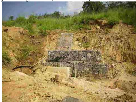
Small landslide behind the gabion wall caused by cutting work (Point No.1)
