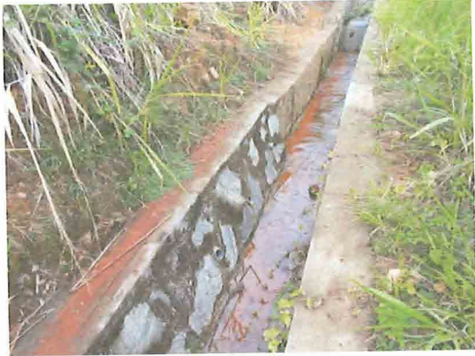
Photo 1: Erosion has been corrected (Loc.2)
