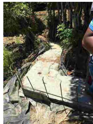
Photo 4.4 Sudden curves of ditch (already corrected )
