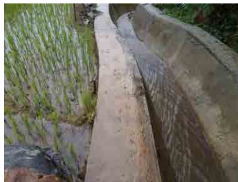
Photo 6: Crack has been corrected. (Loc. 5)
