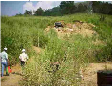
Embankment at the middle of the slope (Point No.1)
