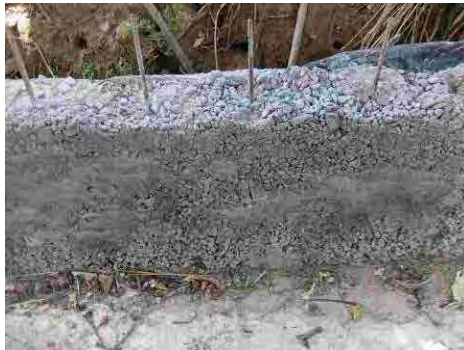
Photo 4.2 Honeycombs of surface drainage ditch (already corrected)
