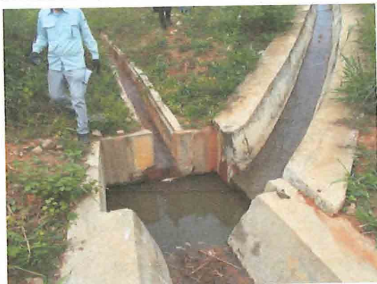
Photo 5: Soils have been removed (Loc.7)
