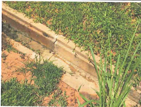
Photo 9: Crack has been corrected (Loc.11)
