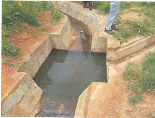
Photo 7: Soils have been removed (Loc.8)
