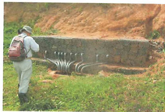
Photo 12: PVC pipe has been repaired (D.P.6)
