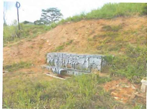
Photo 10: The small slip has been reshaped (D.P.4)
