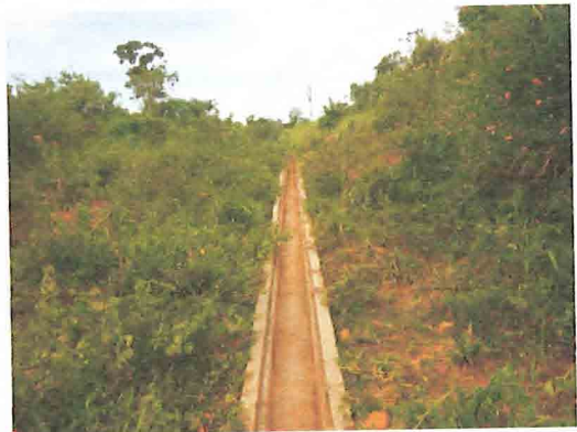
Photo 6: Rocks have been removed (Loc.12)
