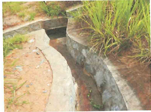
Photo 2: Erosion has been corrected (Loc.1)
