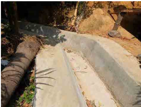
Photo 4.5 Sudden curves of ditch
