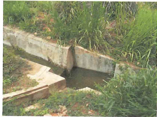
Photo 8: Soils have been removed (Loc.9)
