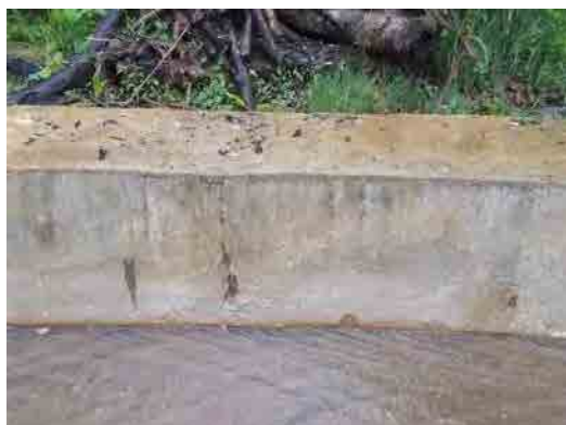
Photo 9: Leakage has been repaired. (Loc. 13)
