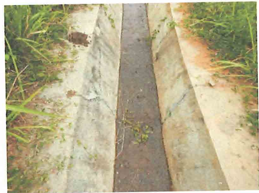
Photo 4: Cracks have been corrected (Loc.5)
