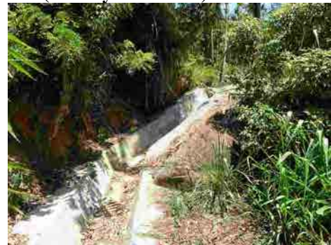
Photo 4.5 Sudden curves of ditch
