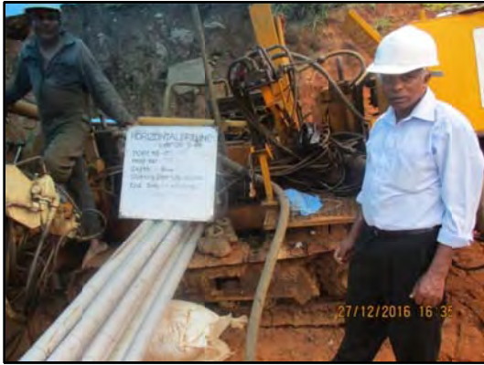
PVC pipes prepared and numbered before installation
