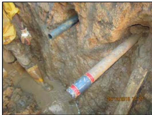
PVC pipes installed in to holes
