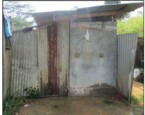
Bathing and washing facility at site
