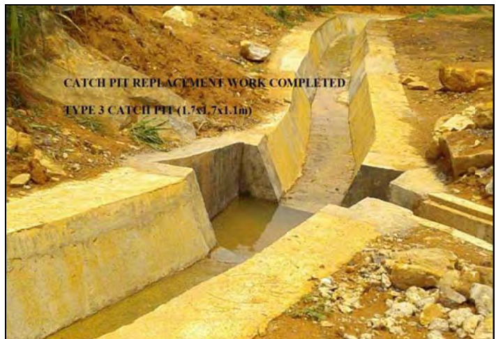
Catch pit type 3 replacement work completed
