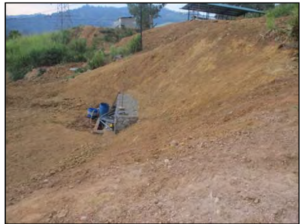
New location 4 after reshaping
