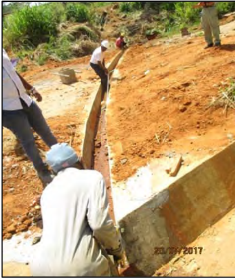
Length of surface drain type E being checked
