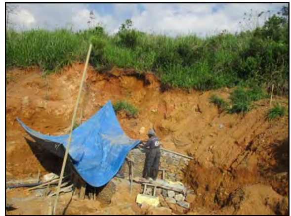
Stone filling behind and beside gabion wall
