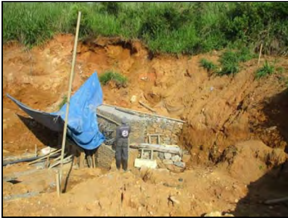
Stone filling behind gabion walls
