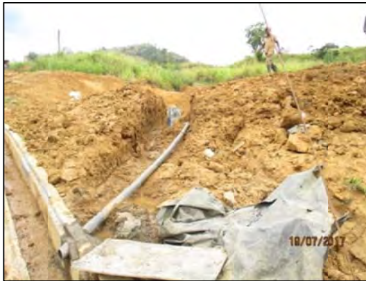
Underground PVC pipe connecting catch pit to the drain
