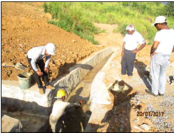
Inspection of additional drains by NBRO
