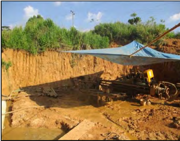
Holes being drilled at location 6
