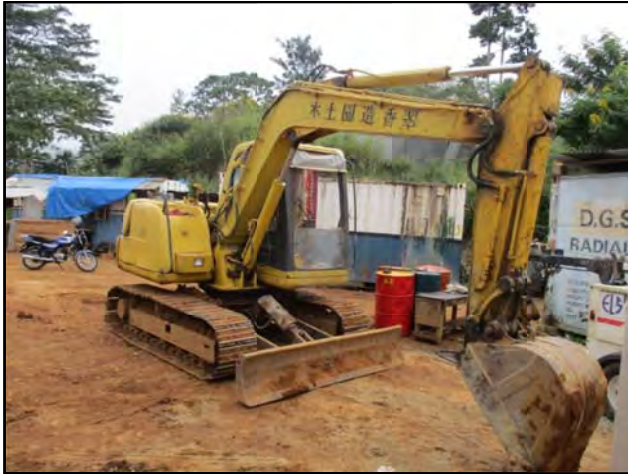
Laboratory, storage facilities, excavator at site
