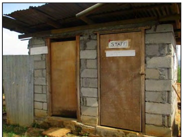
Sanitary facilities at site
