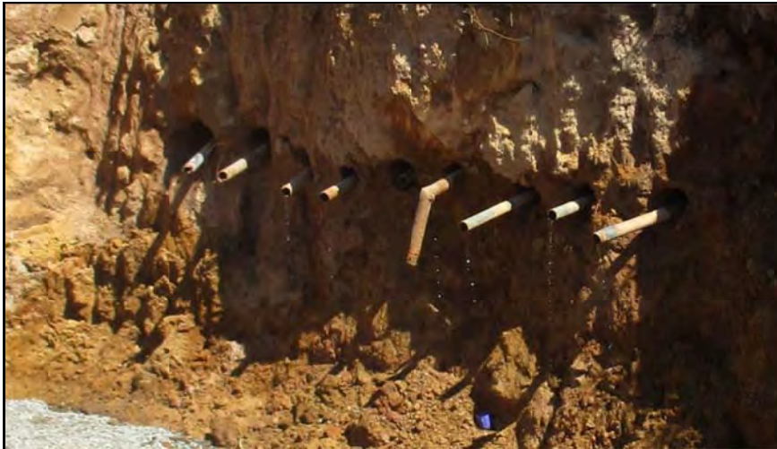
Drilling completed at location 5
