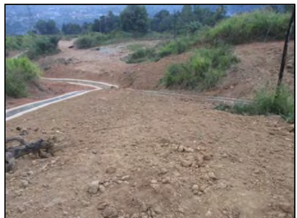
Reshaping around surface drains
