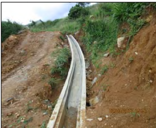
Type E drain (141m)
