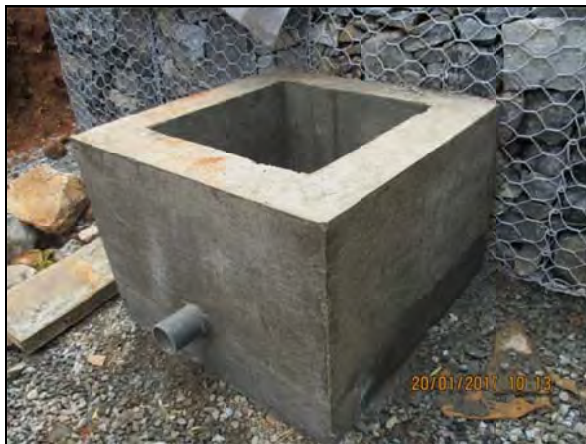
Type 1 catch pit constructed in front of gabion wall
