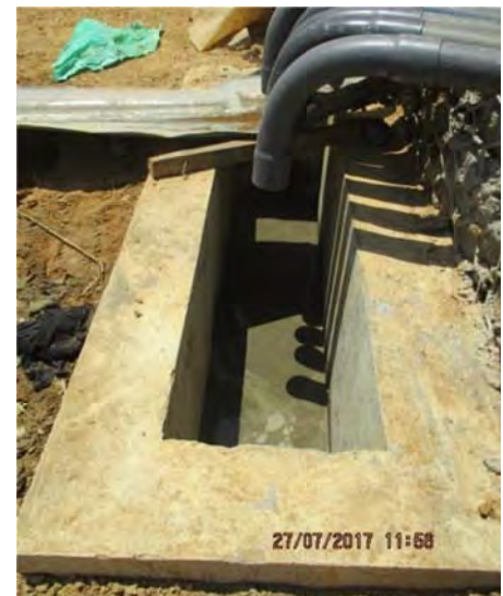
Type 1 catch pit constructed at location 4
