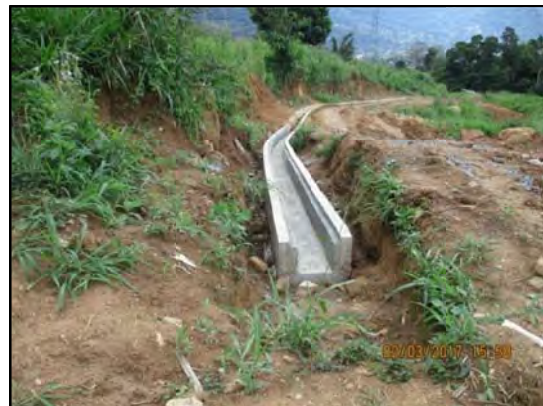
Type E drain (141m) starting point
