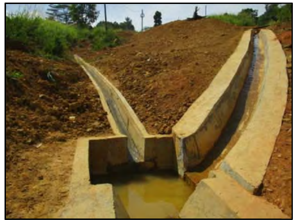
Type E, D and C drains jointing together
