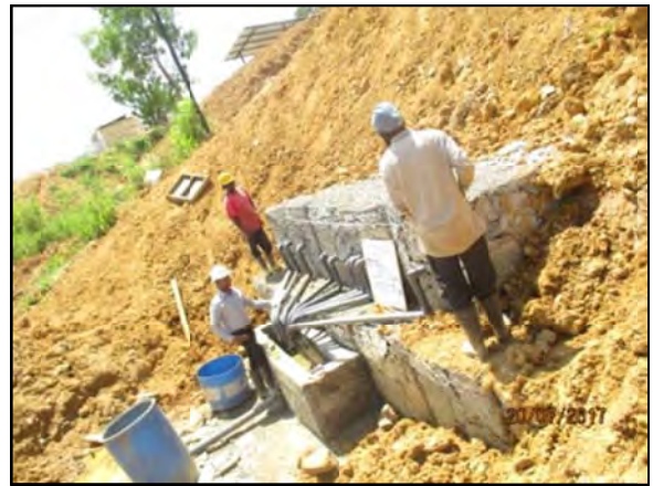
Gabion work completed at location 4
