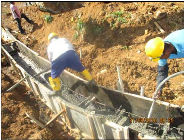
Concrete compacted with poker vibrator
