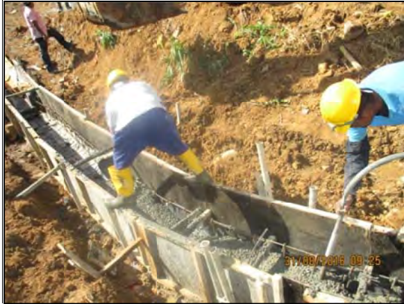
Formwork for concrete drains
