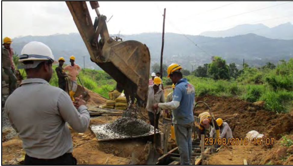
Concreting the surface drains
