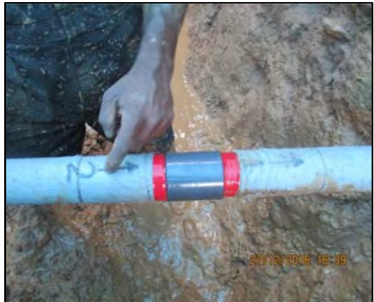
PVC pipes being installed in order
