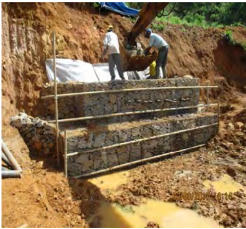
Gabion work at point location 6
