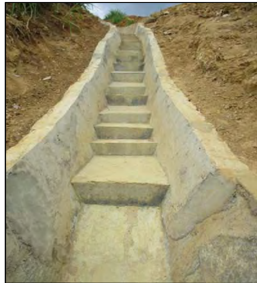
Additional cut off drain
