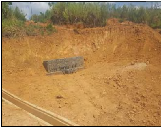
Gabion work at location 5
