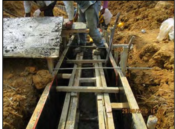
Formwork for concrete drains
