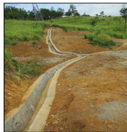
Drains additionally constructed
