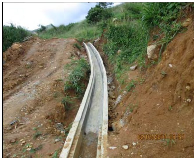
Neat and smooth finish of the drain
