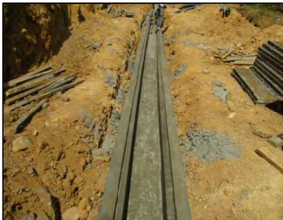
Type E drain when formwork removed
