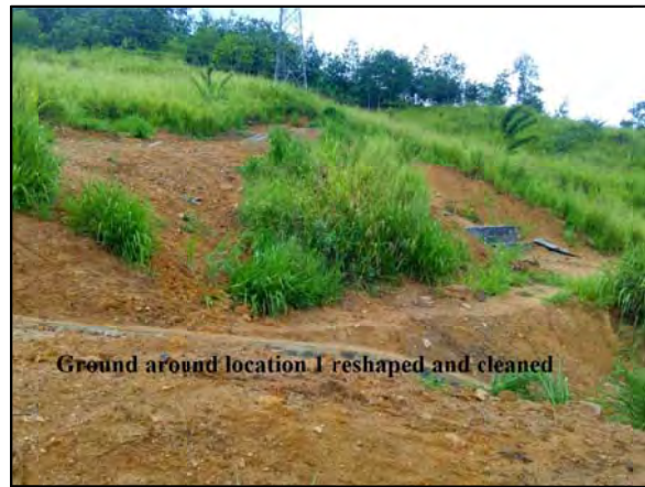
Location 1 after reshaping
