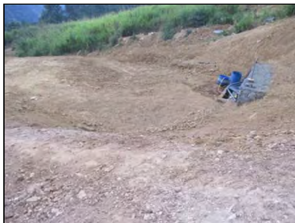
Reshaping completed at new location 4
