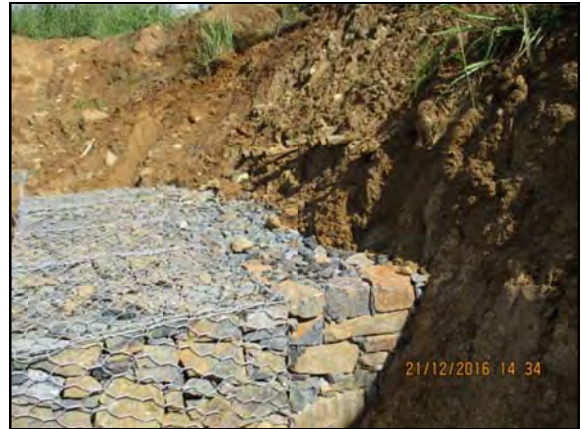
Stone filling behind gabion walls
