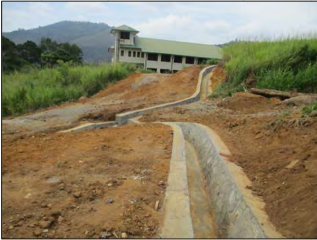
Additional cut off drain
