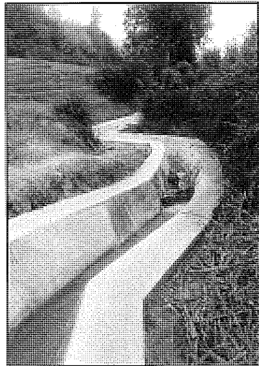
Fig 29: Completed drain section
