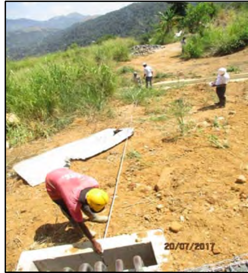
Length of PVC pipes laid underground being checked
