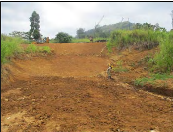
Old location 4 after reshaping
