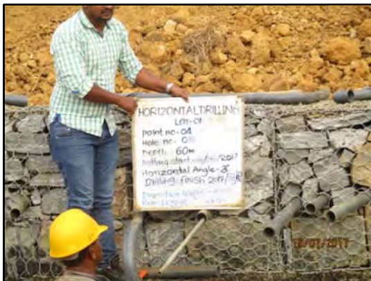
Hole lengths and Gabion work being measured and checked by JICA
