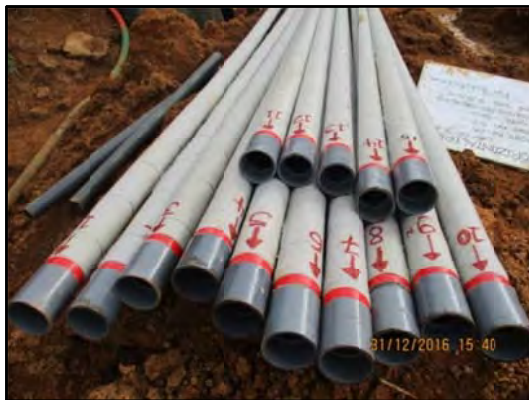
PVC pipes numbered before installation
