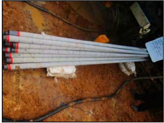
PVC pipes prepared and numbered before installation
