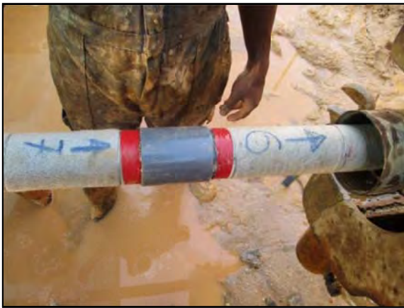
PVC pipes driven into holes through casing
