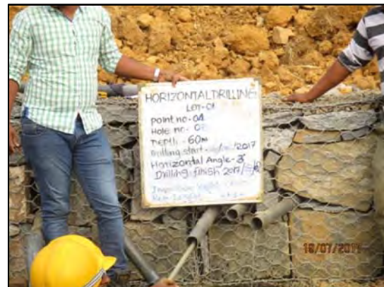
Hole lengths and Gabion work being measured and checked by JICA
