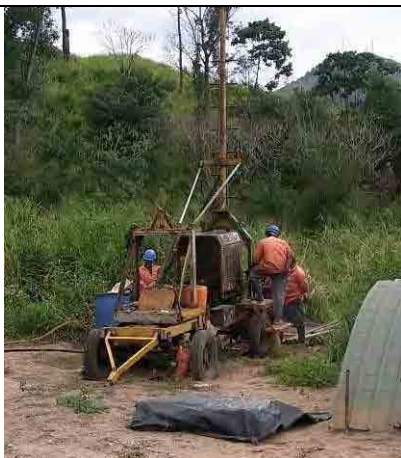
Figure 3.3 Drilling Work at the Site
