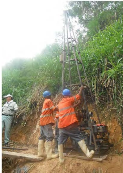
Figure 3.3 Drilling Work at the Site
