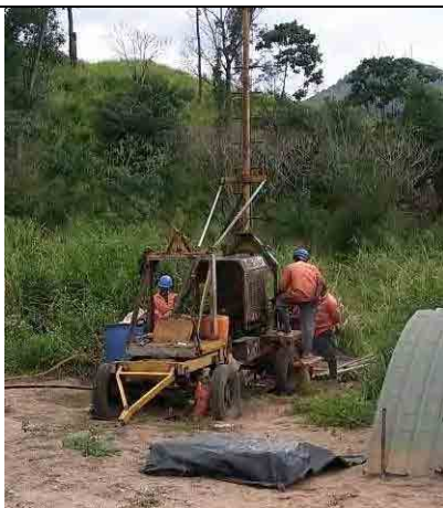
Figure 3.3 Drilling Work at the Site
