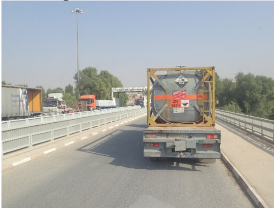
Bridge over the Jordan river (SHB)
