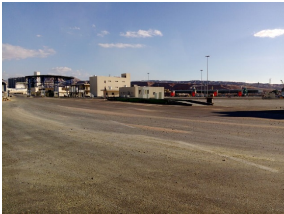
New container terminal at Aqaba Port
