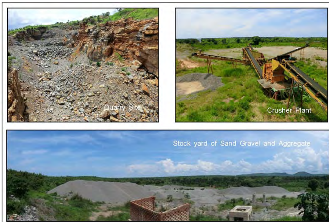
Photo 2.2.4.1-5 Quarry Site at Ilagala
