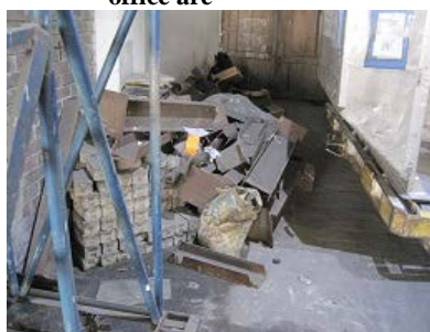
Photo 2.4-121 Inside the sorting area
