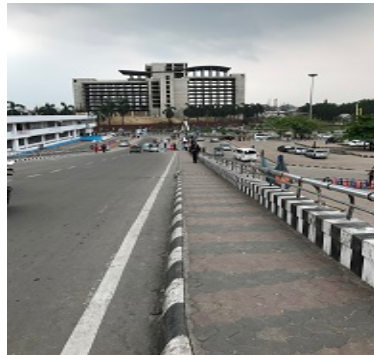
Photo 2.4-7 Pathway and Slope that connects to Departure Floor
