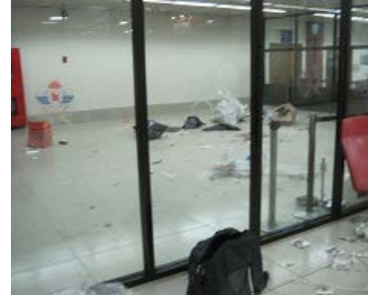
Photo 2.4-88 Lost baggage storage room where the garbage is scattered
