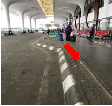
Photo 2.4-6 Level Difference at the Curbside
