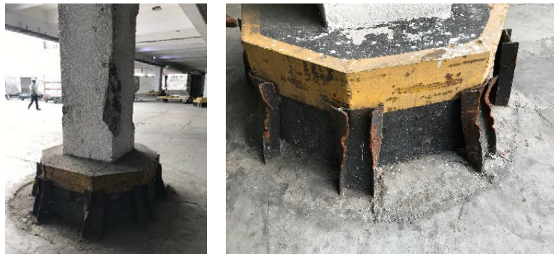
Photo 2.4-54 Damaged Pillars
