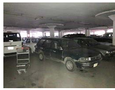
Photo 2.4-99 Inside Multistory Parking Lot
