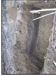
Temporary Sedimentation Pit
