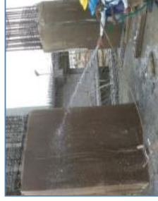
Use of Gunny bags for curing during construction
