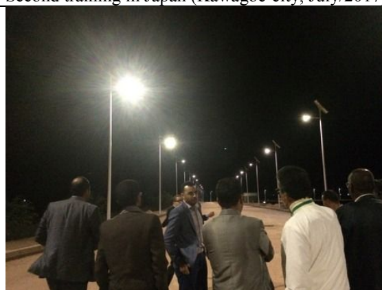
Visit site of solar power light (November/2017)
