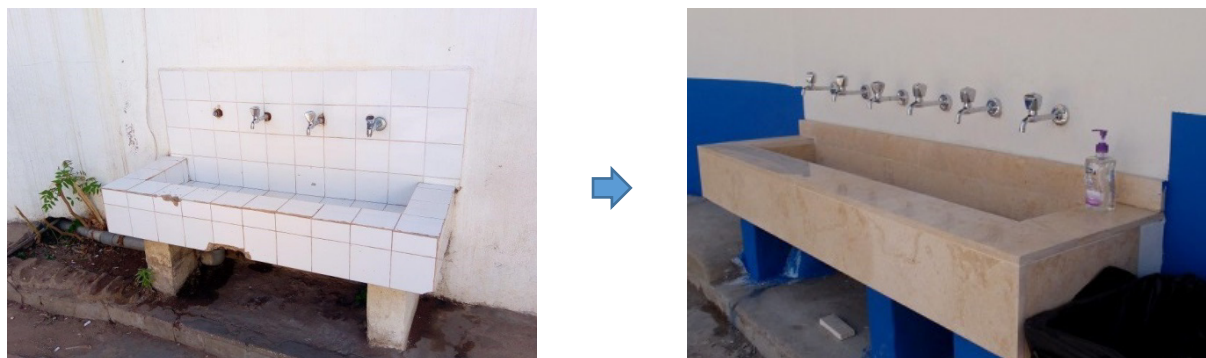
Zouk Mosbeh School: Renovation of washing basin in the play ground
