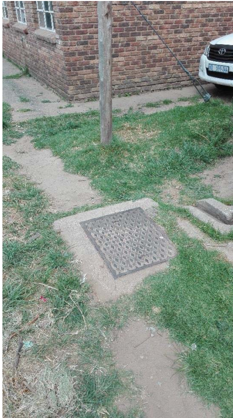
Plate 3 : Example of manhole for possible sewerage / storm water disposal system existing on site.
