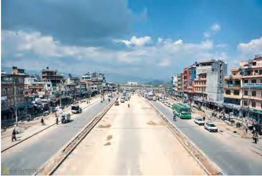
Photo 3.6-2 Ring Road Expansion
