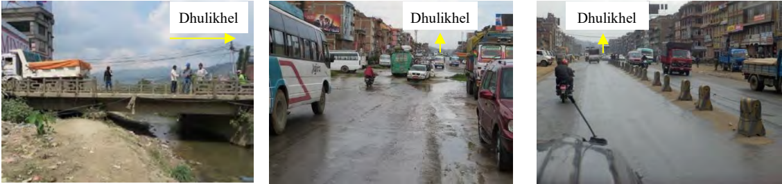
(1) 17m Long bridge at Punyamati River
