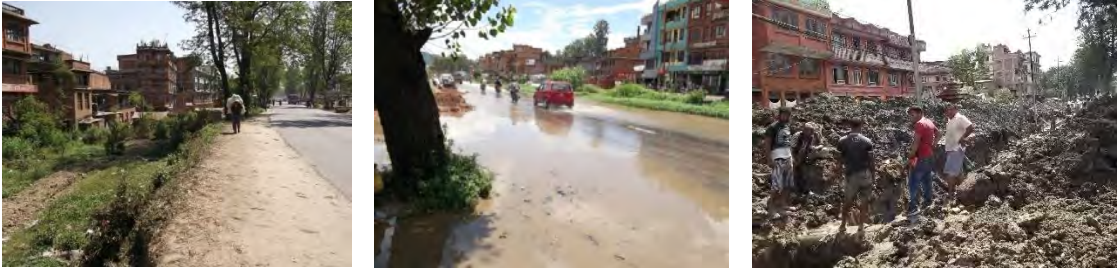
(1) Elevation difference at Suryabinayak (2) Inundation at Jagati (3) Installation of Temporary Drainage by DOR
