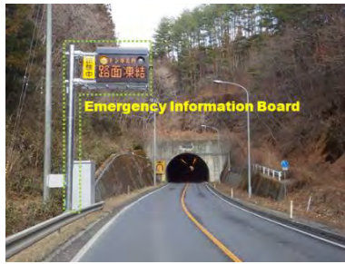
Emergency Information Board
