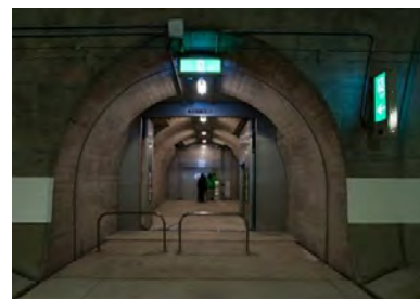
Evacuation Route (Evacuation Connection Tunnel)
