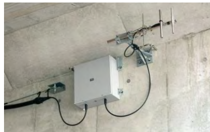
Photo 11.6-10 Wireless Radio System
