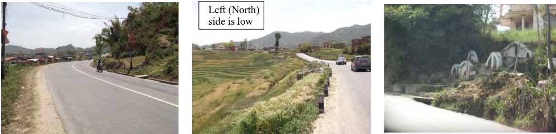
(1) Sharp curve (accident prone area)
