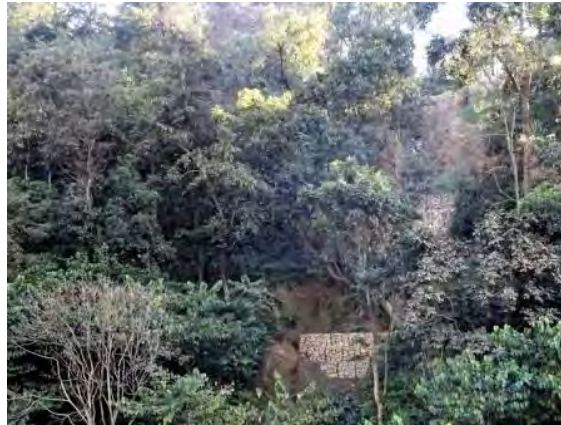
Figure 8.2-3 Collapse Prevention Retaining Wall
