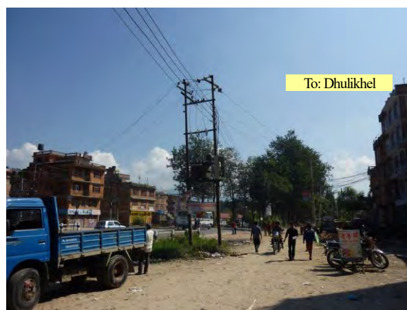
Photo-8: City of Suryabinayak (Telegraph pole and steel poles inside ROW)
