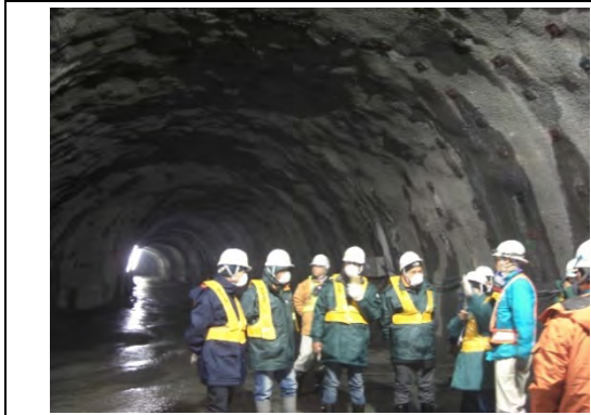
Pic-5 : Sinkuzakai Tunnel
