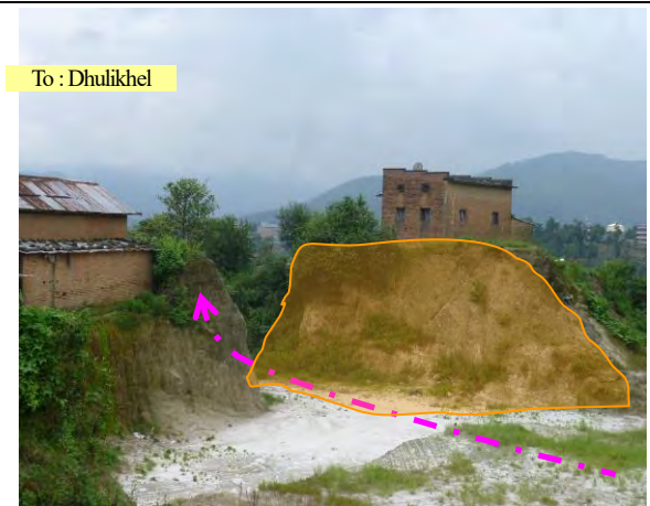
Photo-21 : Cut slope near Dhulikhel
