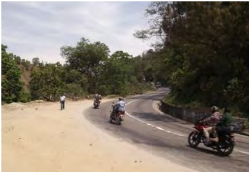
(4) Sharp Curve with Steep Grade near Sanga Pass
