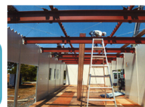
Construction work by Pre-fabricated System Architecture
