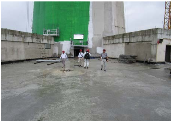
Rooftop of Tower Base
