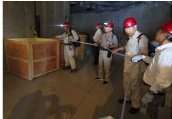
Confirmation of route for carrying in cables in Tower Base
