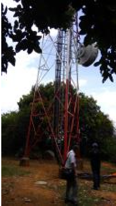
Antenna Tower in Badulla
