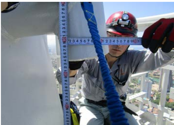
Measurement working at T1 Section
