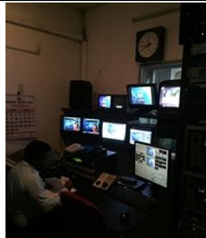
Control facility (EAP)
