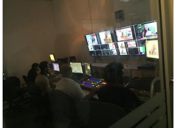
Control facility (Derana TV)
