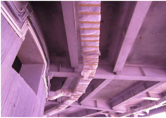
Fire prevention section in Tower House
