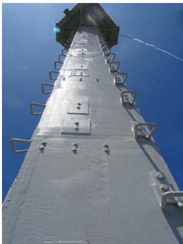
Antenna installation part
