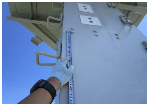
Measurement of holes for bolts at antenna installation part
