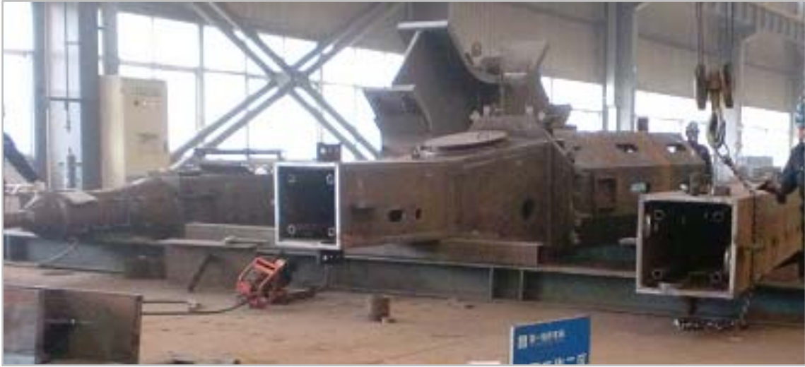
64. Photo of T1 Section as of inspection in China
