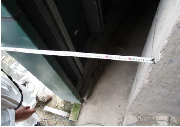
Measurement of part for laying cables at Micro platform
