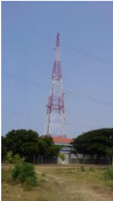
Antenna tower in Jaffna
