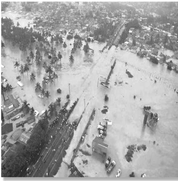
Plate 3: Poor drainage system caused the flooding of Morogoro trunk road in 2017
