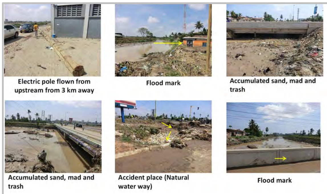
Figure 5.1.37 Jangwani Bridge on Morogoro Road on 9 March 2017, 10:30
