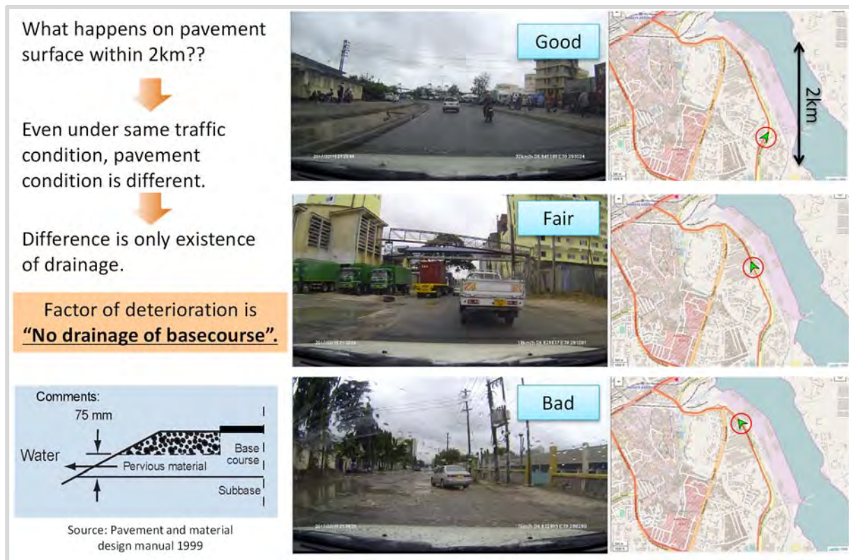
Figure 5.1.39 Observation on Pavement Structure
