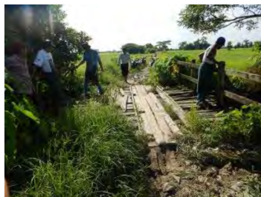
Figure 3-1-7 Timber decked bridge
