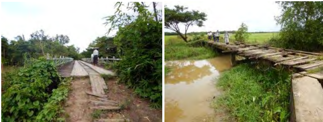
Figure 3-1-9 Timber decked bridges at Sa Bai Kone Village Tract
