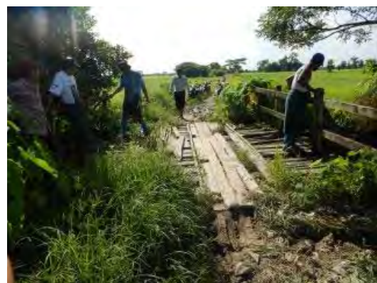
Figure 3-1-7 Timber decked bridge
