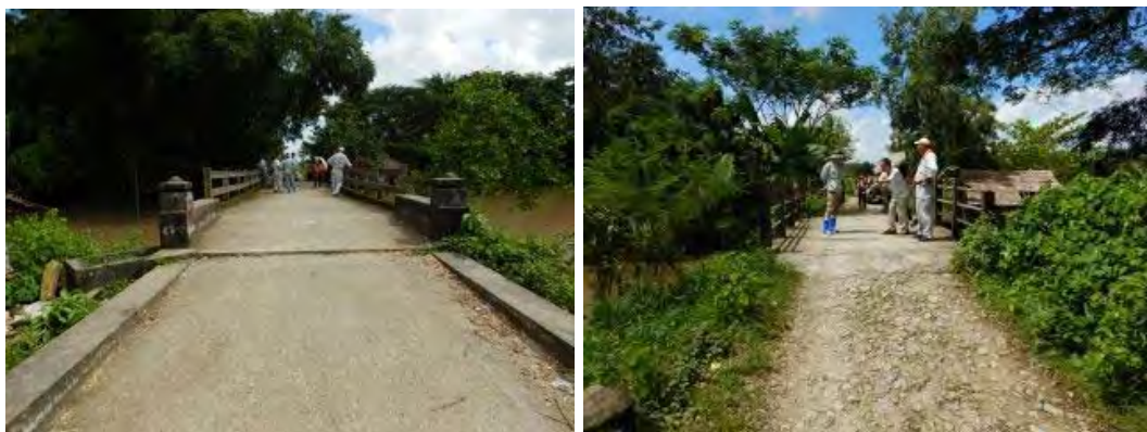
Figure 3-1-11 Existing concrete bridge in Tha Kan Wa Village Tract
