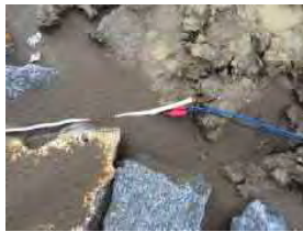
Temporary electrical wiring in Lagunbyin NOT acceptable
