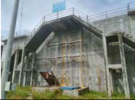
Remedial work of water leakage, 29 Jan. 2017
