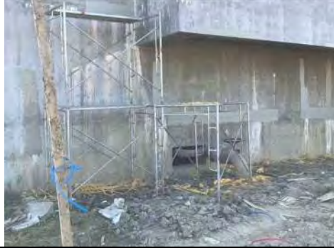
Remedial work of water leakage, 05 Feb. 2017
