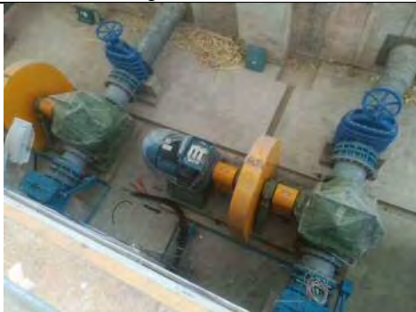
Wiring work, 21 Jan. 2017
