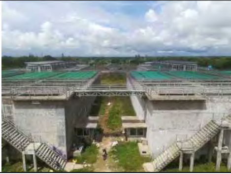
Remedial work of water leakage, 12 Oct. 2017
