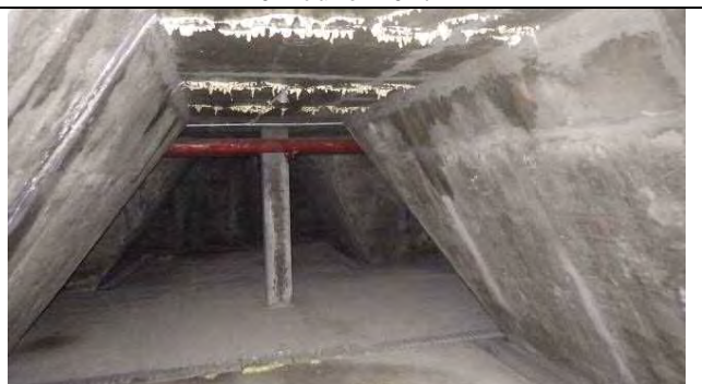
Remedial work of water leakage, 20 Sep. 2017
