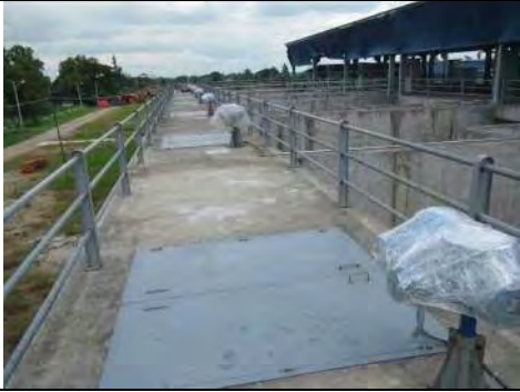
Drain valve, 28 Sep. 2016
