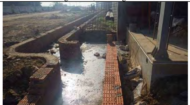
Drainage ditch, 21 Feb. 2017
