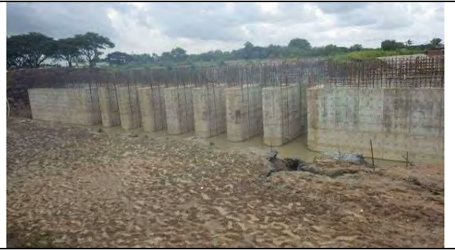
Intake gate, 04 Sep. 2015
