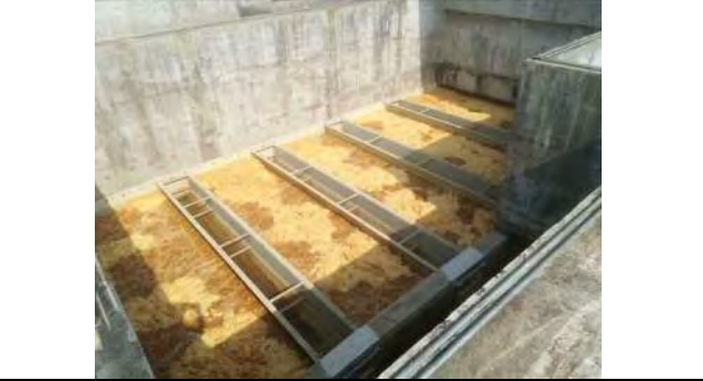
Test of back washing, 17 Jan. 2018
