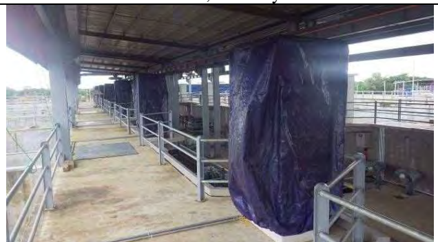
Control panel, 21 July 2016
