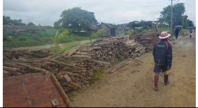
Removal of temporary material, 05 Oct. 2015
