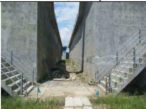
Drainage ditch, 28 Sep.2 2016
