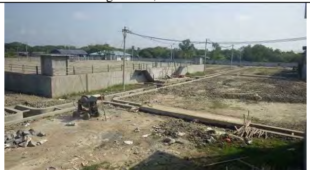
Drainage ditch, 26 April 2017
