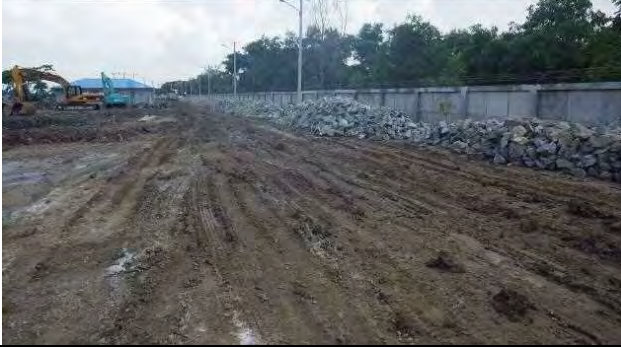
Service road, 02 June 2015
