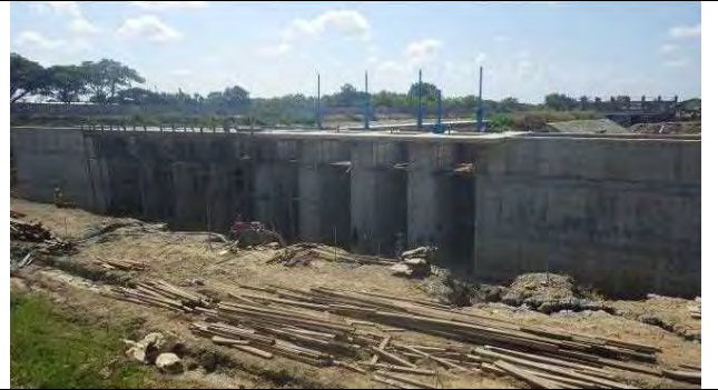
Intake gate, 05 Jan. 2015
