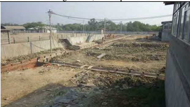
Drainage ditch, 21 March 2017
