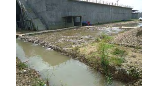
Drainage ditch, 25 Aug. 2016
