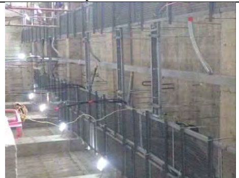
Wiring work, 27 Feb. 2017
