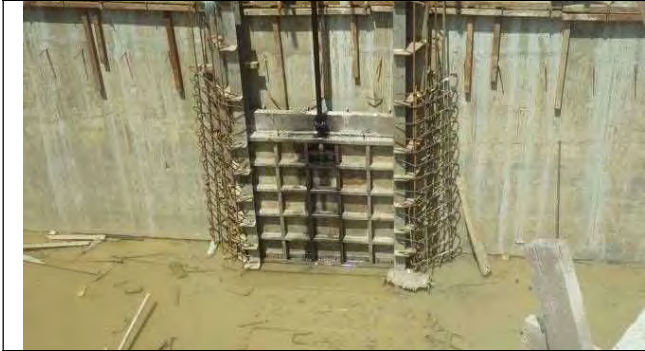
Intake gate, 29 Sep. 2015
