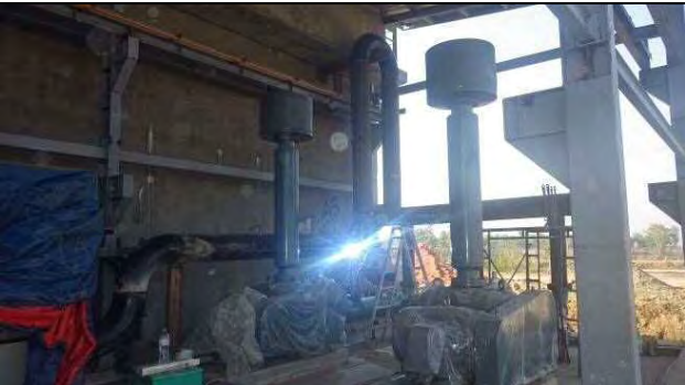
Change of air pipe route, 21 Feb. 2017
