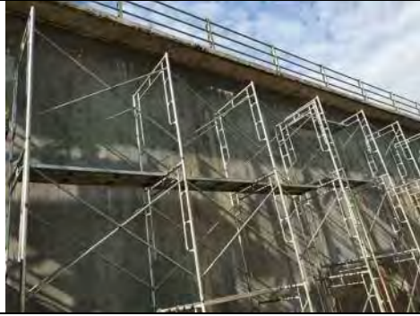
Remedial work of water leakage, 07 Jan. 2017
