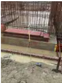
Temporary electrical wiring in Lagunbyin NOT acceptable
