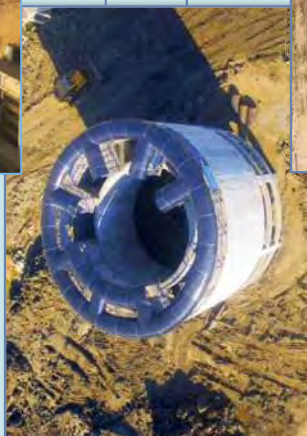
Dividing Well Super Structure
