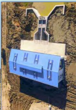
Lift Pumping Station
