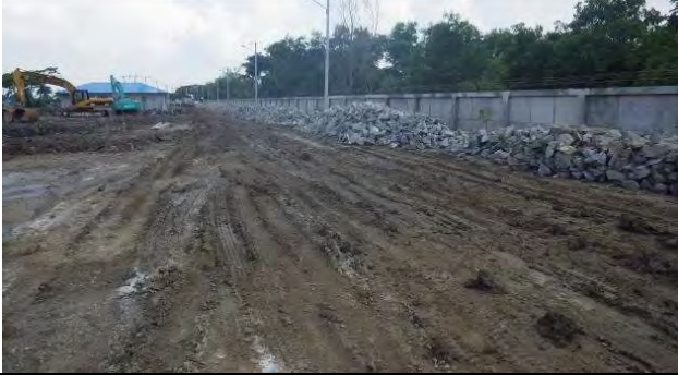
Service road, 02 June 2015
