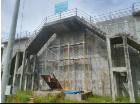
Remedial work of water leakage, 29 Jan. 2017
