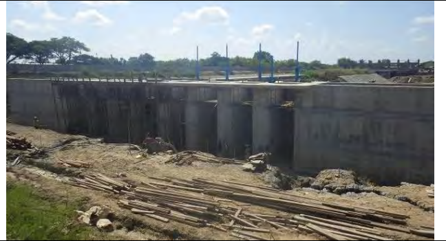
Intake gate, 05 Jan. 2015
