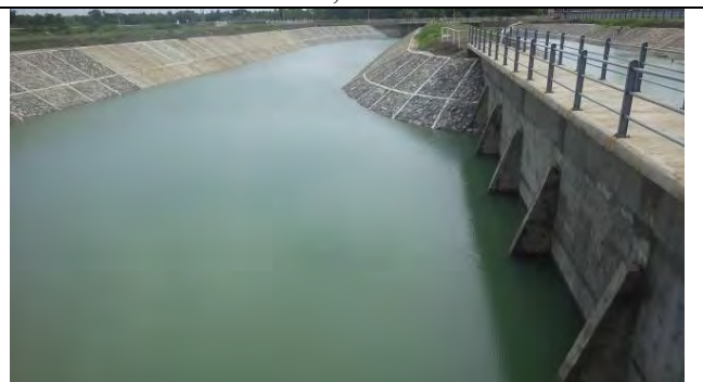
Grit chamber, 09 June 2016
