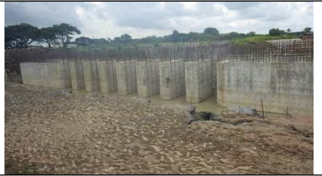
Intake gate, 04 Sep. 2015
