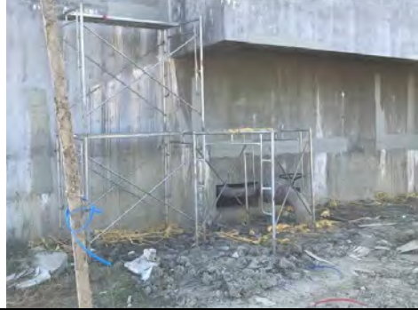
Remedial work of water leakage, 05 Feb. 2017
