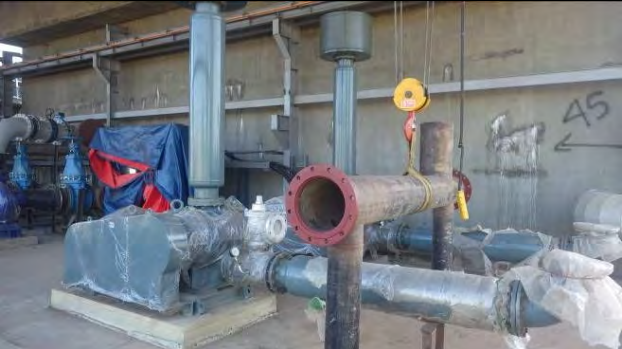
Change of air pipe route, 03 Jan. 2017
