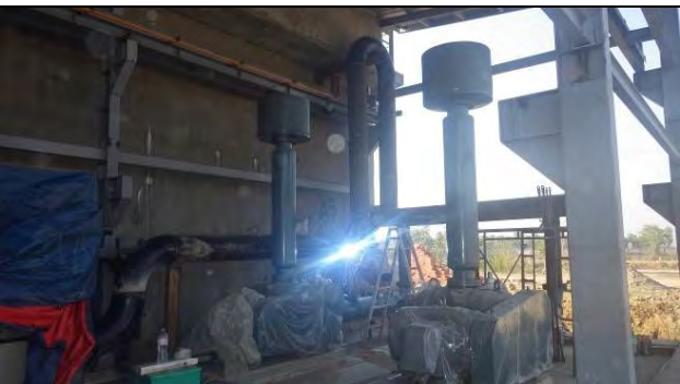
Change of air pipe route, 21 Feb. 2017
