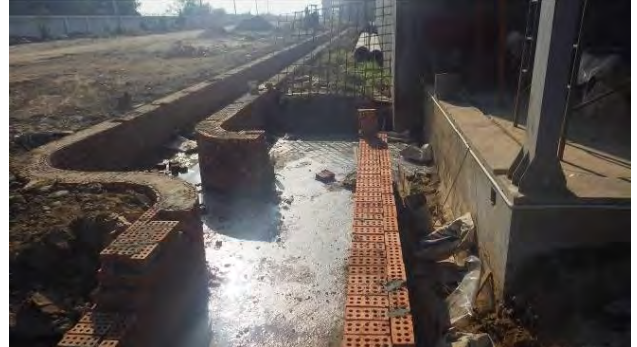
Drainage ditch, 21 Feb. 2017
