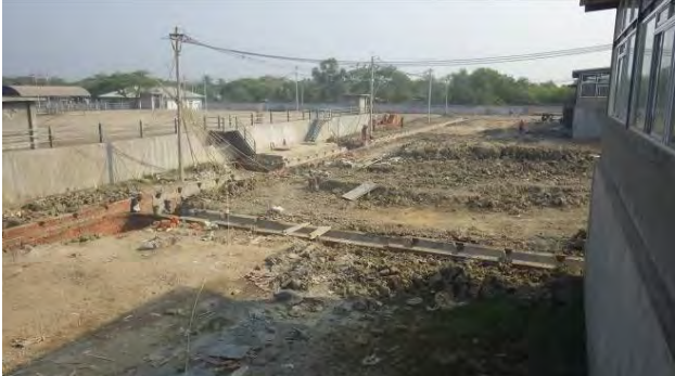
Drainage ditch, 21 March 2017
