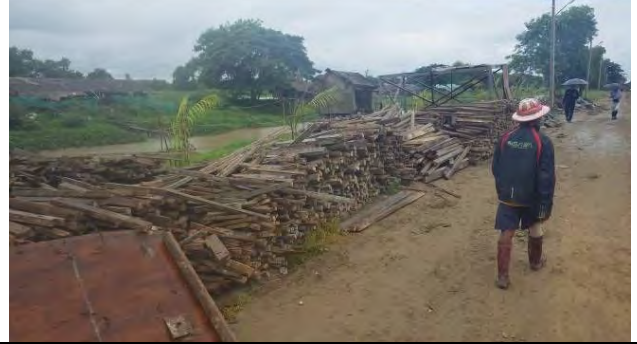
Removal of temporary material, 05 Oct. 2015
