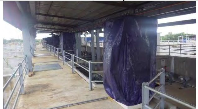
Control panel, 21 July 2016
