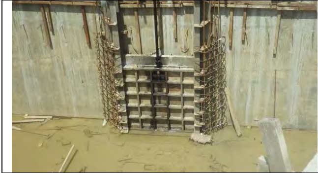
Intake gate, 29 Sep. 2015
