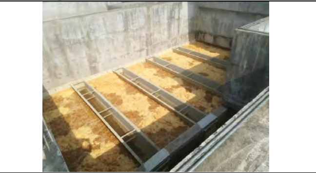
Test of back washing, 17 Jan. 2018
