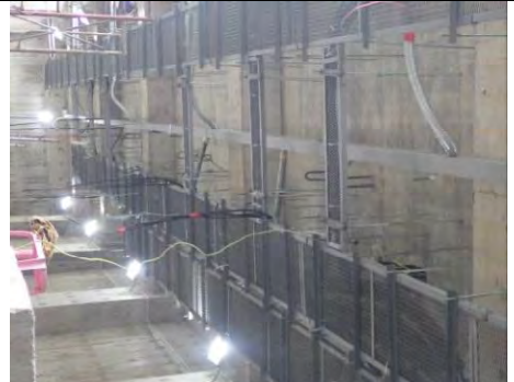
Wiring work, 27 Feb. 2017
