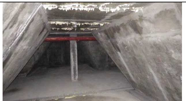
Remedial work of water leakage, 20 Sep. 2017
