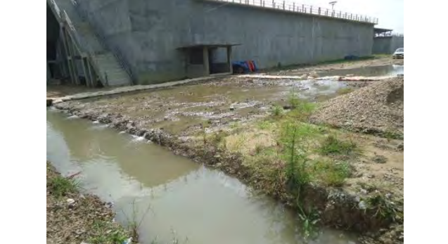
Drainage ditch, 25 Aug. 2016
