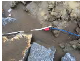
Temporary electrical wiring in Lagunbyin NOT acceptable
