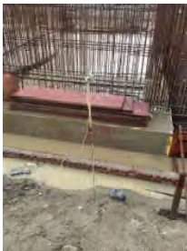
Temporary electrical wiring in Lagunbyin NOT acceptable
