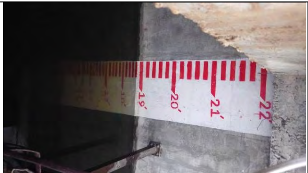
Watertightness Tests for Clear Water Tank (31 Aug 2016)
