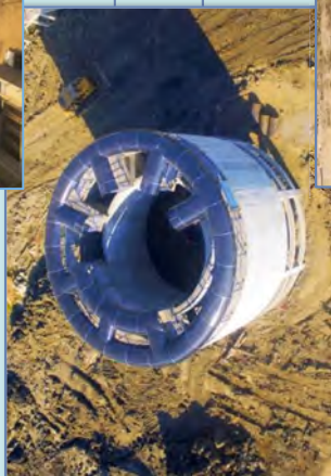
Dividing Well Super Structure
