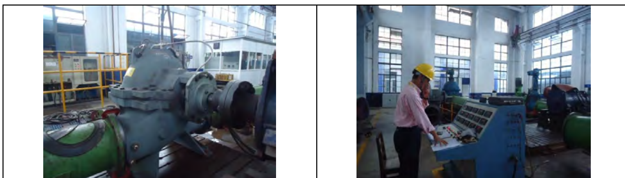
Factory Inspection: Lift Pumps (09 Jul 2015)
