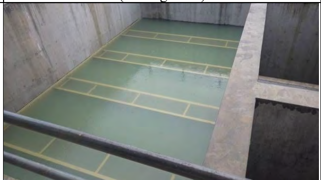
Watertightness Tests for Filter Tank (28 Oct 2016)
