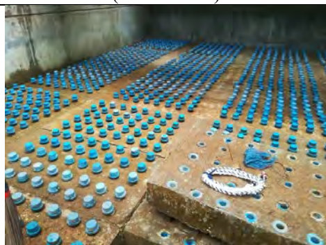
Strainers Condition (29 Aug 2017)
