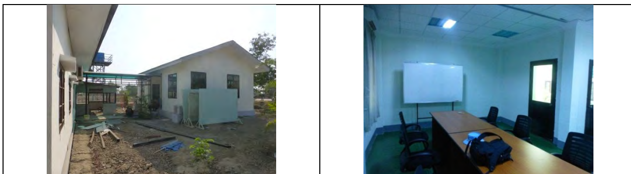
Office in the Lagunbyin WTP (20 Mar 2014)
