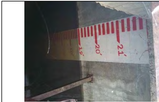
Watertightness Tests for Clear Water Tank (28 Jul 2016)
