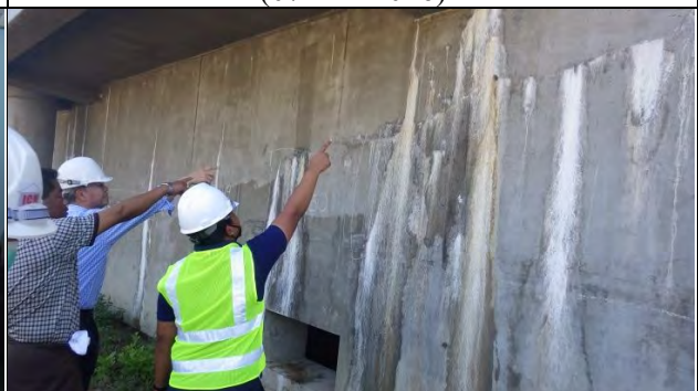
Test Construction (14 Jan 2017)
