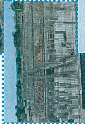
The construction work For Super Structure of Clear Water Reservoiř
