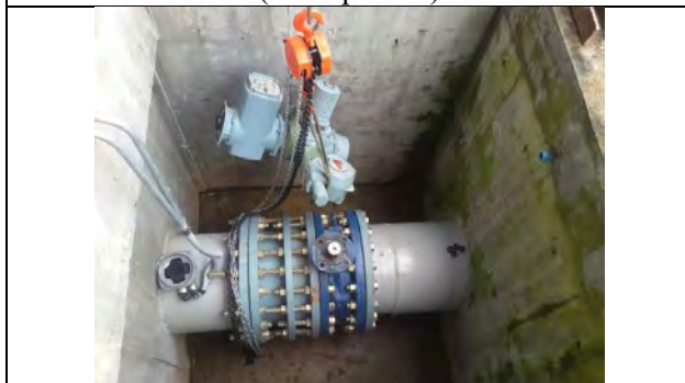
Repair Work of Inlet Valve (28 Jul 2017)
