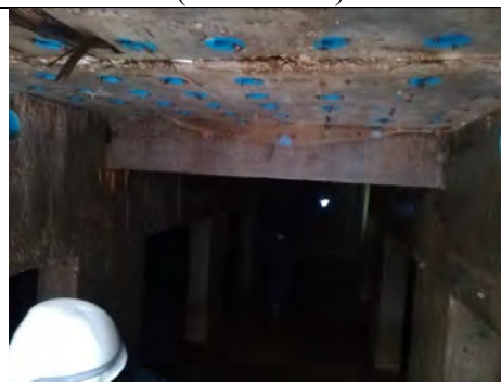
Joint Inspection under Filter Tank (29 Aug 2017)
