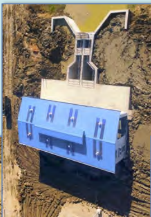
Lift Pumping Station
