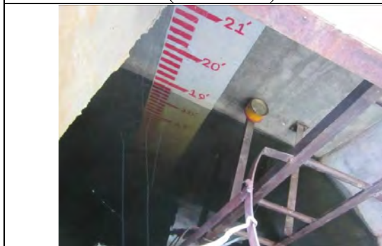
Watertightness Tests for Clear Water Tank (28 Sep 2016)
