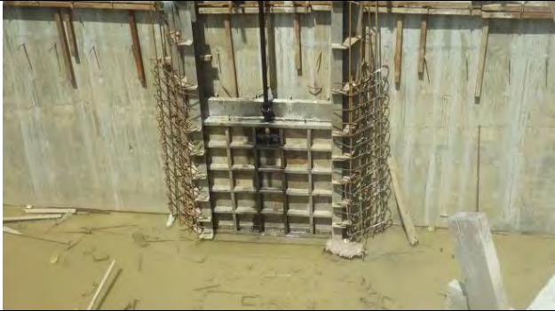
Intake gate, 29 Sep. 2015
