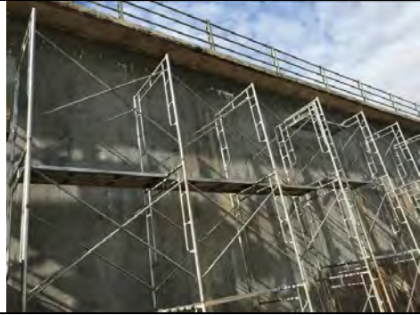
Remedial work of water leakage, 07 Jan. 2017
