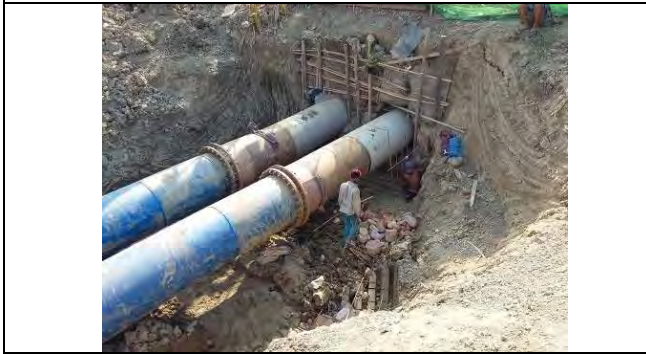
Railway crossing, 05 April 2016
