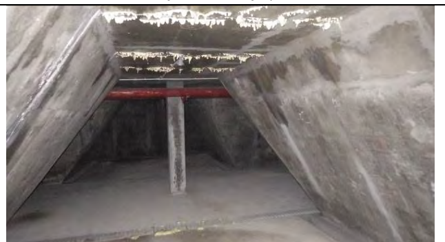
Remedial work of water leakage, 20 Sep. 2017
