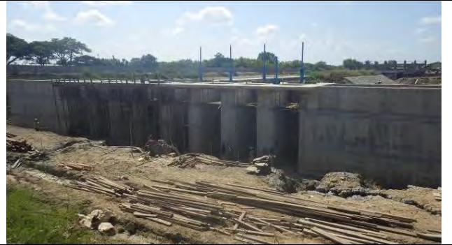
Intake gate, 05 Jan. 2015
