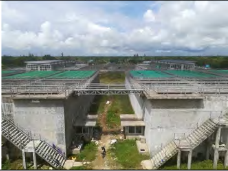
Remedial work of water leakage, 12 Oct. 2017
