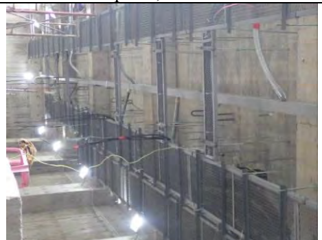
Wiring work, 27 Feb. 2017
