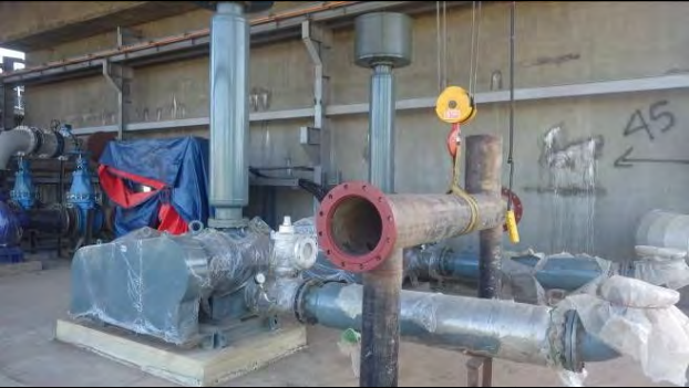
Change of air pipe route, 03 Jan. 2017
