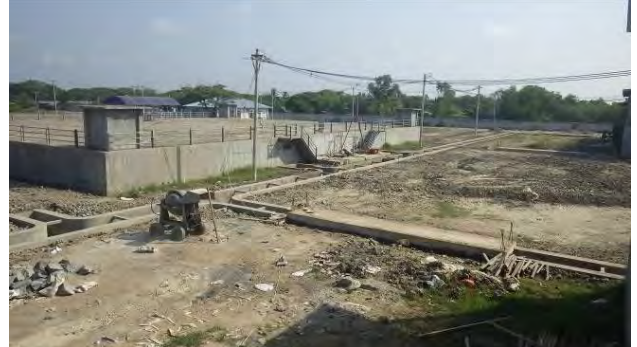
Drainage ditch, 26 April 2017
