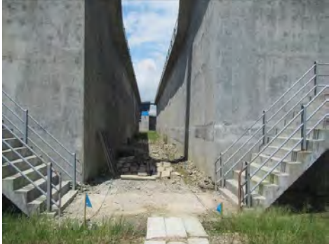
Drainage ditch, 28 Sep.2 2016
