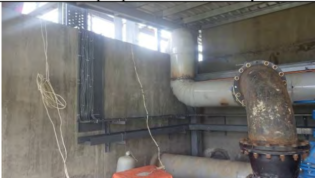
Pipe route, 21 July 2016
