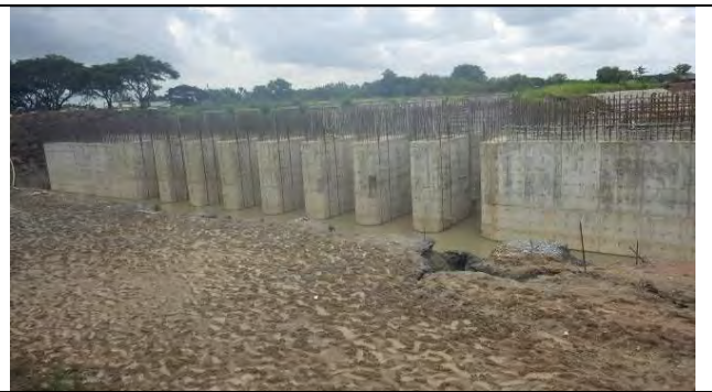
Intake gate, 04 Sep. 2015
