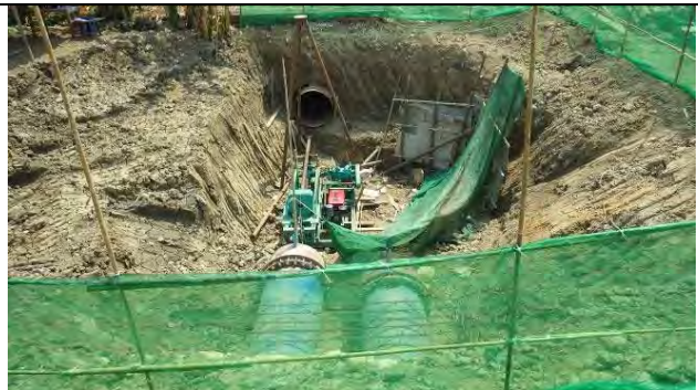
Railway crossing, 03 March 2016
