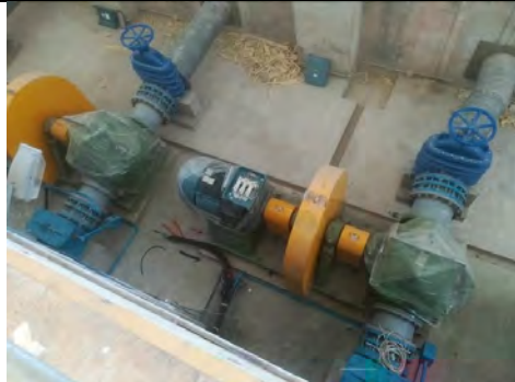
Wiring work, 21 Jan. 2017
