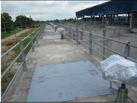
Drain valve, 28 Sep. 2016
