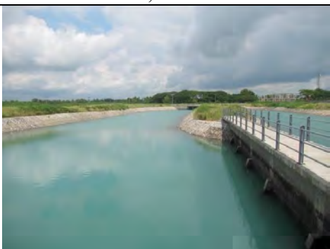
Grit chamber, 28 Sep. 2016
