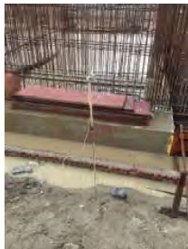
Temporary electrical wiring in Lagunbyin NOT acceptable
