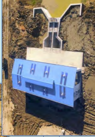
Lift Pumping Station
