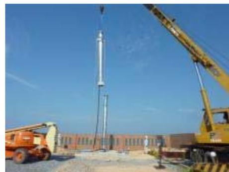
Horizontal level on the top of the tower was measured by level meter and adjusted with wires of 4 corners.
