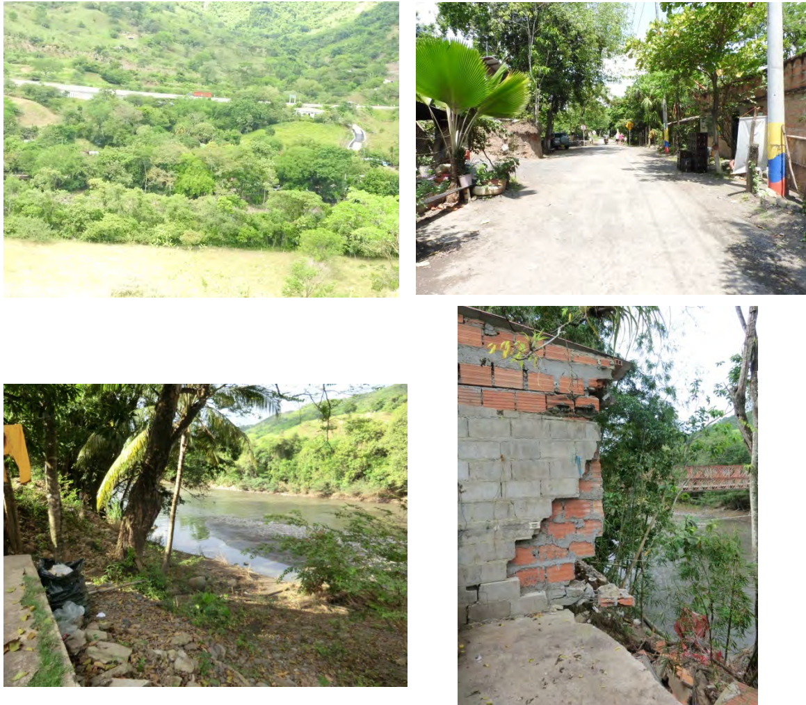
Figure 1.2.1 Proximity of Rio Negro and the Houses in El Dindal
