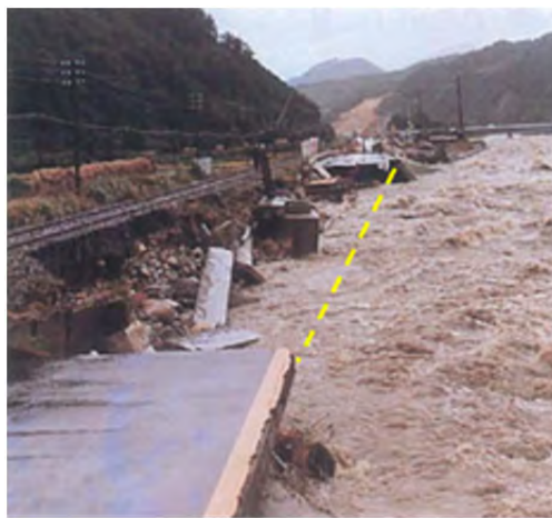
Photo Bank Erosion (Sendai River),1979
