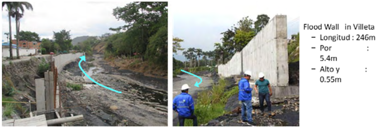
Figure 1.1.3 Flood Wall in Villeta Municipality
