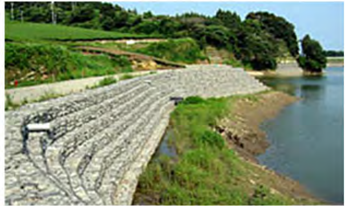
Figure 1.2.4 Structure of Gabions for Shore Protection
