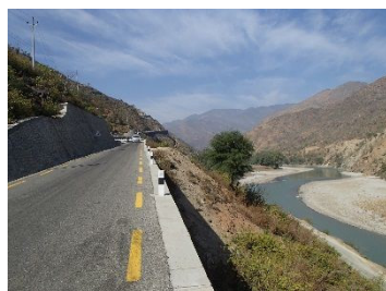
No settlements around Station 11+620 (Distant view)
