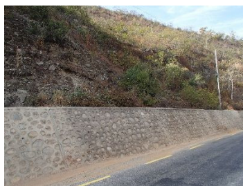
Utility pole on the mountain side above Station 15+520
