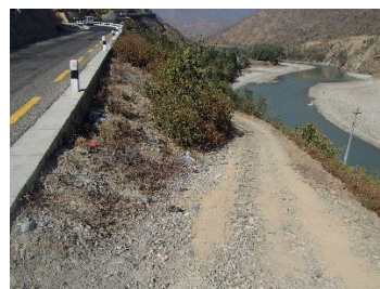
Entrance of unpaved road in the vicinity Station 11+620
