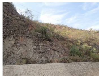
No settlements on the mountain side above Station 15+520
