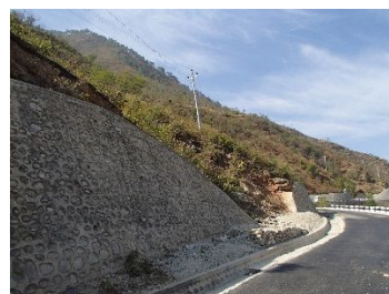
No settlement on the mountain side above Station 11+620
