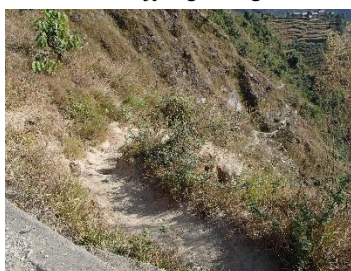
Footpath from Station 17+400 to Khopikharka
