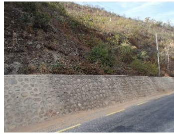
Utility pole in the mountain side above Station 15+520
