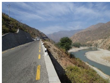
No Settlement around Station 11+620 (Distant view)
