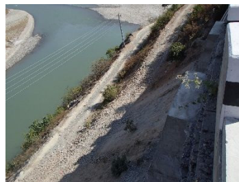
Unpaved road and Utility Pole lie below Station 11+620
