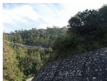
No Settlement in the mountain side above Station 33+695
