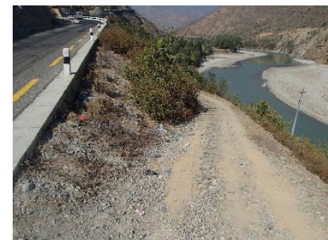
Entrance of unpaved road in the vicinity Station 11+620
