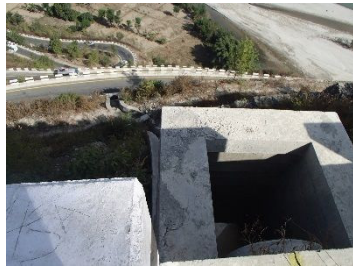
Water Drainage Facility lie below Station 15+520
