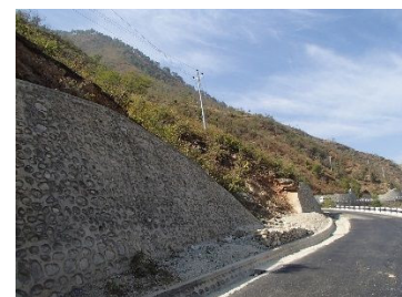
No Settlement in the mountain side above Station 11+620
