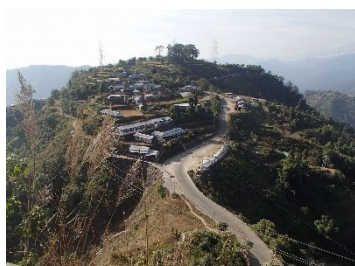
Station 17+400 and Dhungre Bhanjyang village
