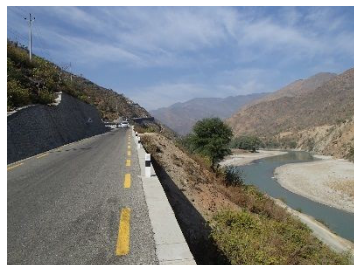
No Settlement around Station 11+620 (Distant view)
