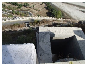
Water Drainage Facility lie below Station 15+520
