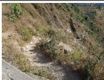
Footpath from Station 17+400 to Khopikharka
