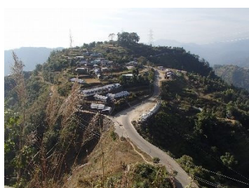
Station 17+400 and Dhungre Bhanjyang village
