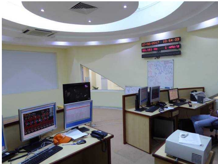
Television in center displays the current grid's diagram. The operators in the cockpits are supervising the grid condition. The clock, frequency and display enabling to display the fault messages are set on the wall
