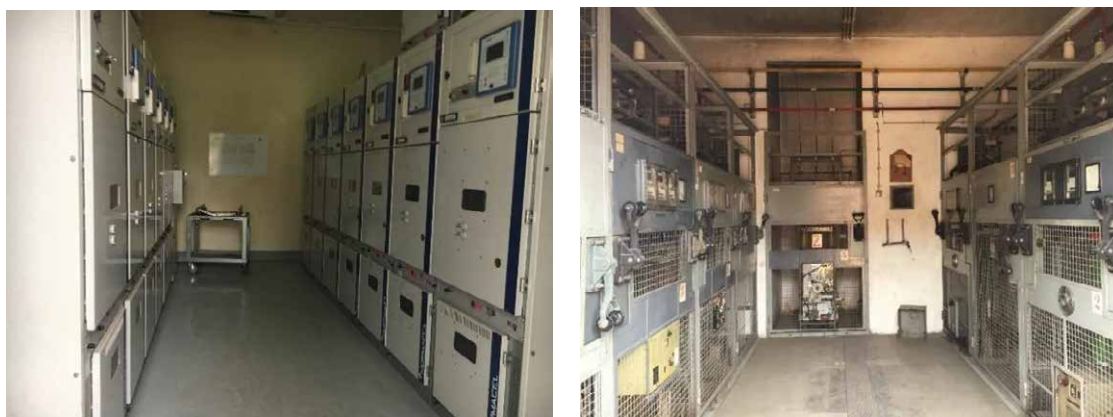
Figure 7.1-5 Inside of PS (Left: Remote operation type, Right: Manual operation type)
