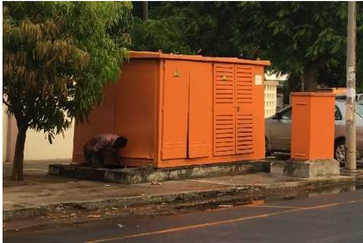
Figure 7.4-2 Transformer for underground line (315kVA)
