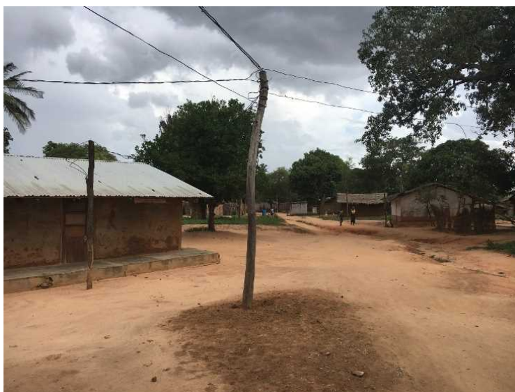
Figure 7.7-2 Non-standard connection of distribution line
