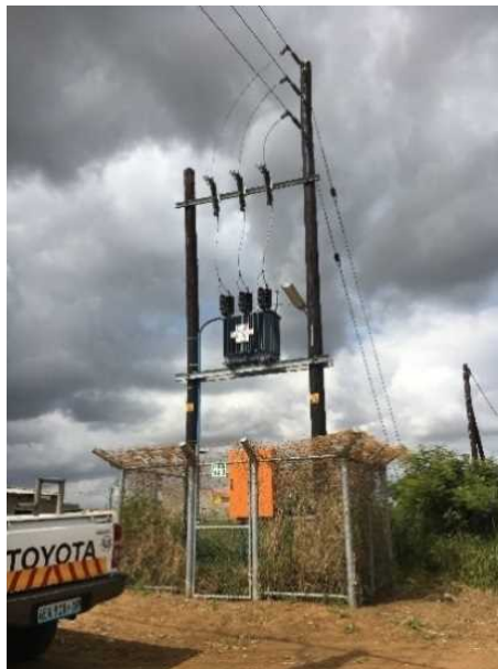
Figure 7.4-1 Transformer for overhead line (100kVA)
