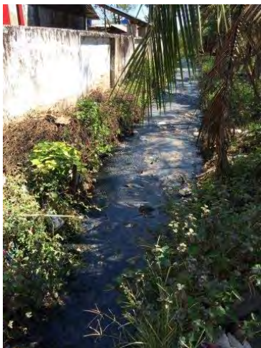
Trench around factories
