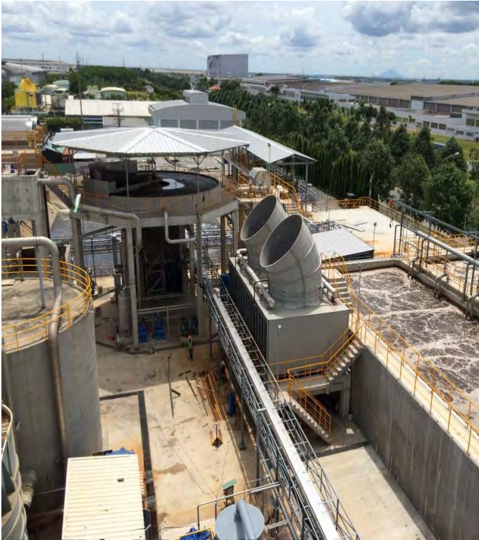
WWTP for PAPER FACTORY Capacity: 8,500 CMD
