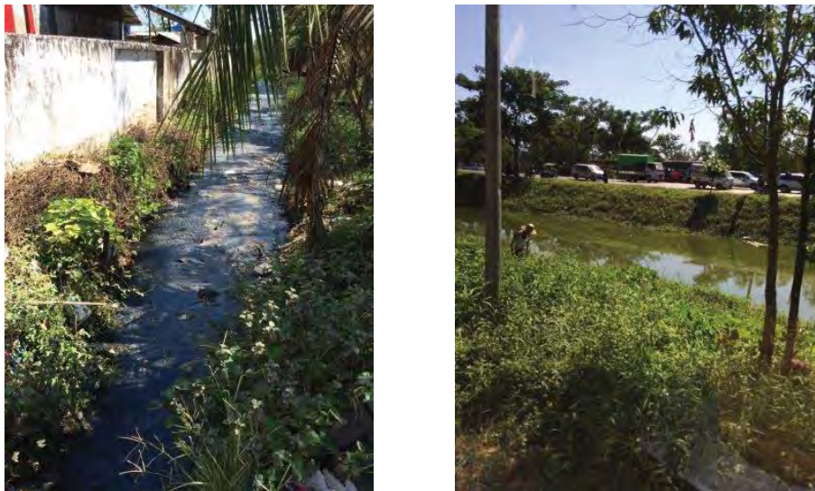
Trench, Creek at outside of factories.
