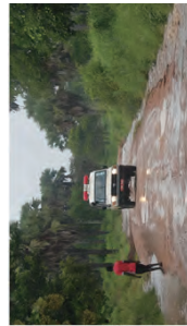
Trenches along the road become like rivers which makes difficult to travel: especially on sections water overflows.
